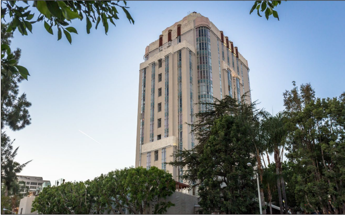
Figure 22: 8358 Sunset Boulevard, 2015. This building is a designated example of the Art Deco style that is individually listed in the National Register, California Register, and as a West Hollywood Cultural Resource (Tony Coelho, City of West Hollywood).
