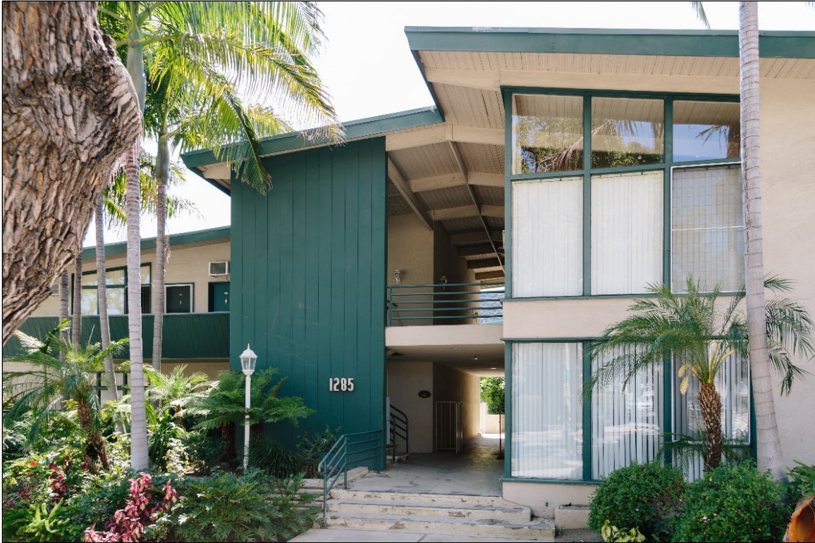
Figure 24: The Fountain Lanai (1285 Sweetzer Avenue), 2015. This building is a designated example of the Mid-Century Modern style that is individually listed as a West Hollywood Cultural Resource (Tony Coelho, City of West Hollywood).
