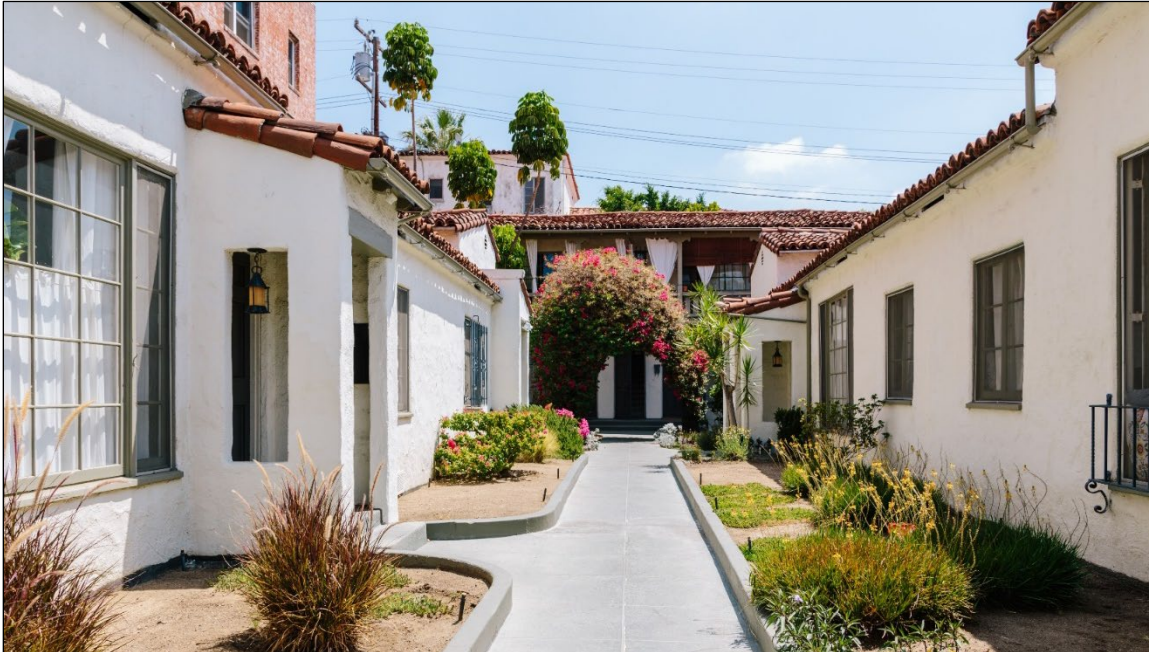
Figure 16: 1230-32 Flores Street, 2015. This building is a designated example of the Spanish Colonial Revival style in West Hollywood. It is listed locally as a contributor to the Courtyard Thematic District (Tony Coelho, City of West Hollywood).
