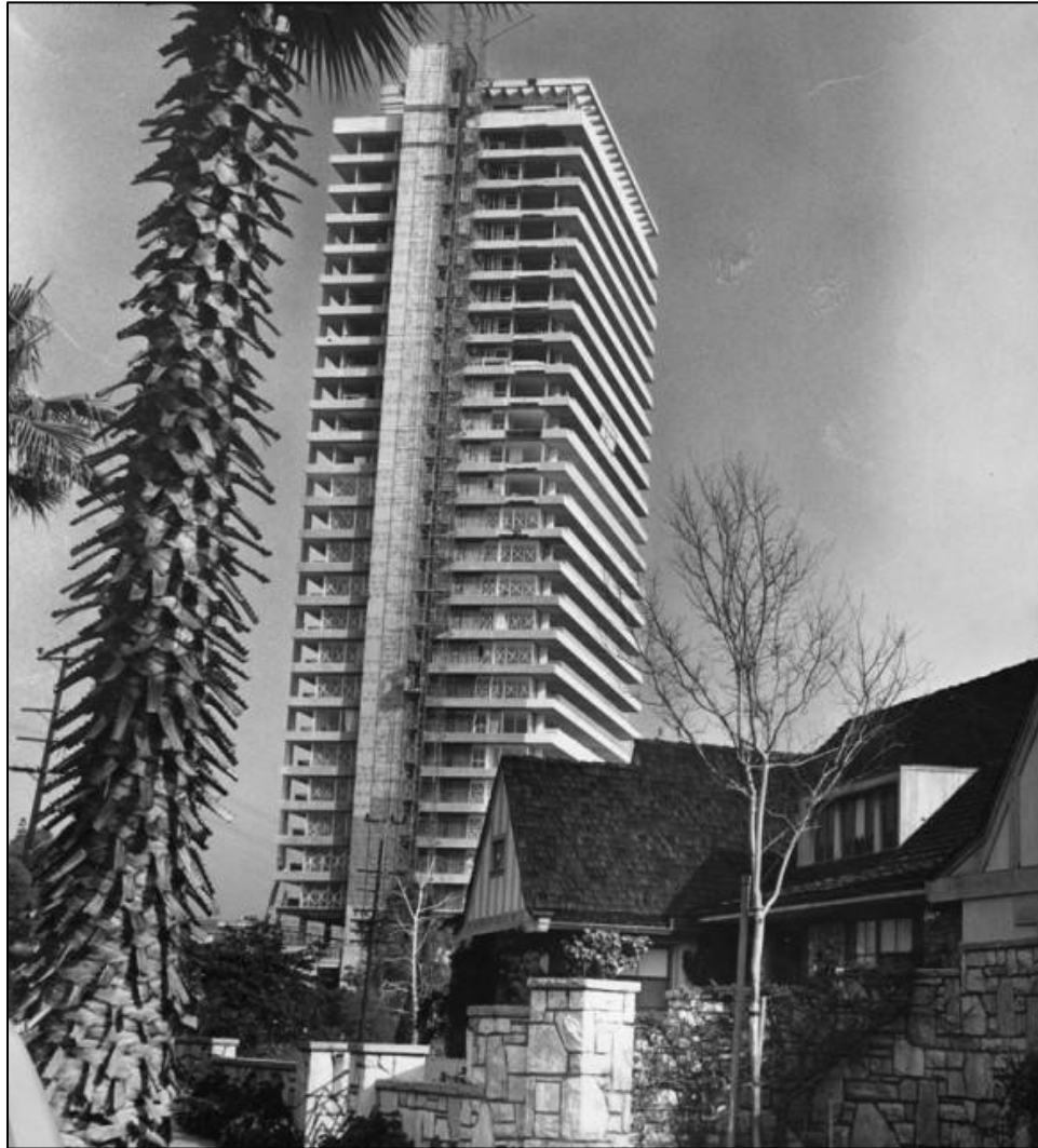
Figure 12: View of Sierra Tower, near Sunset Boulevard and Doheny Drive, under construction c. 1965. (Los Angeles Public Library Digital Collections)
