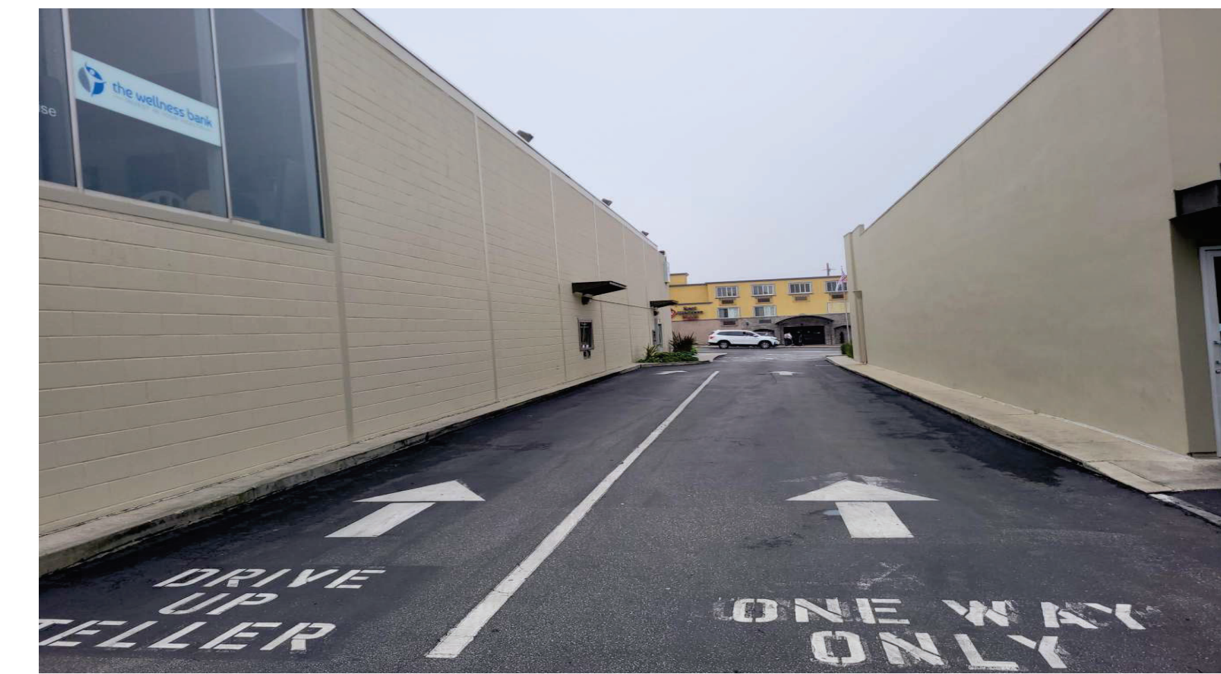
NORTH EXISTING EXTERIOR
