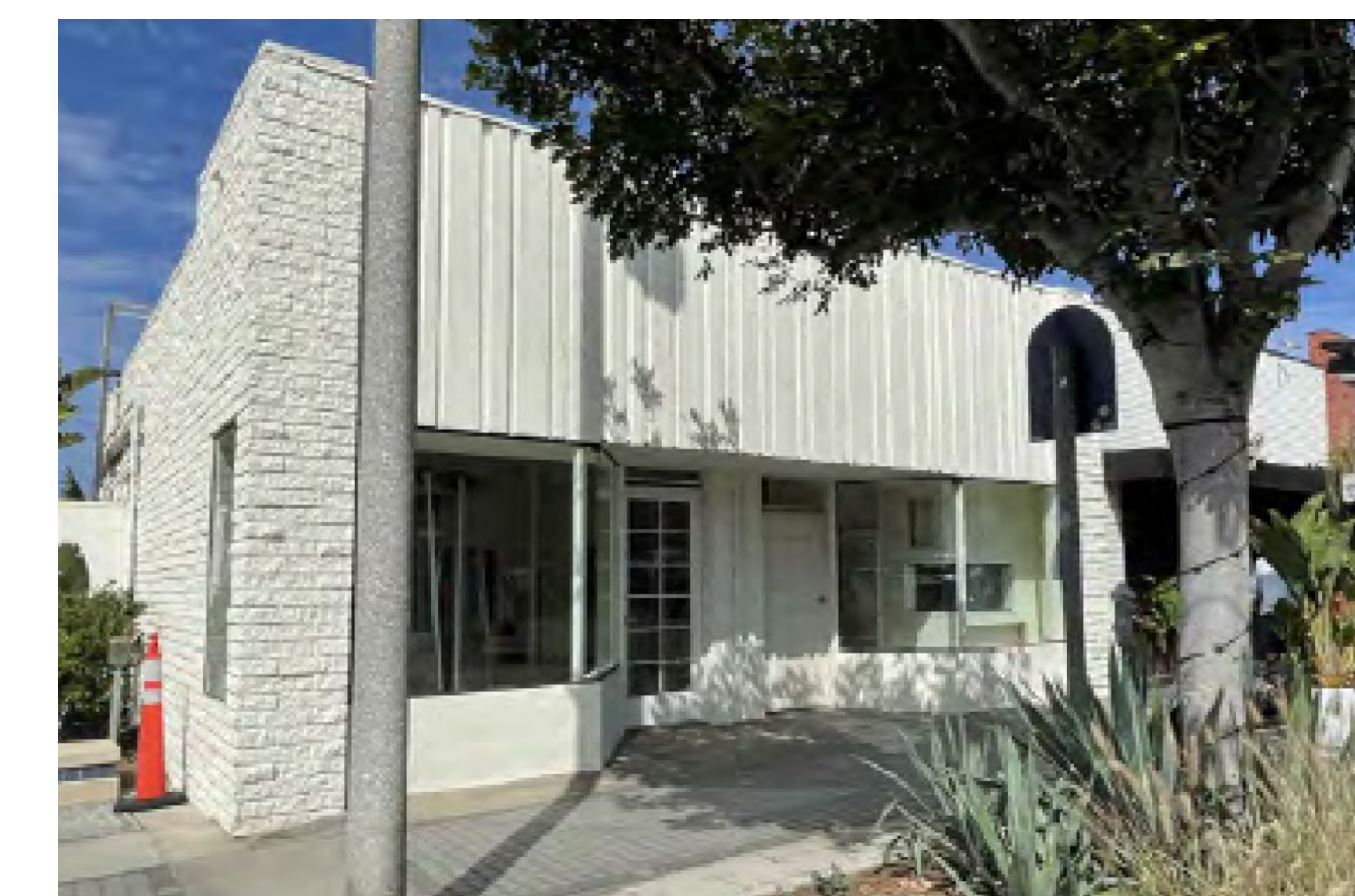
EXISTING STORE FRONT
