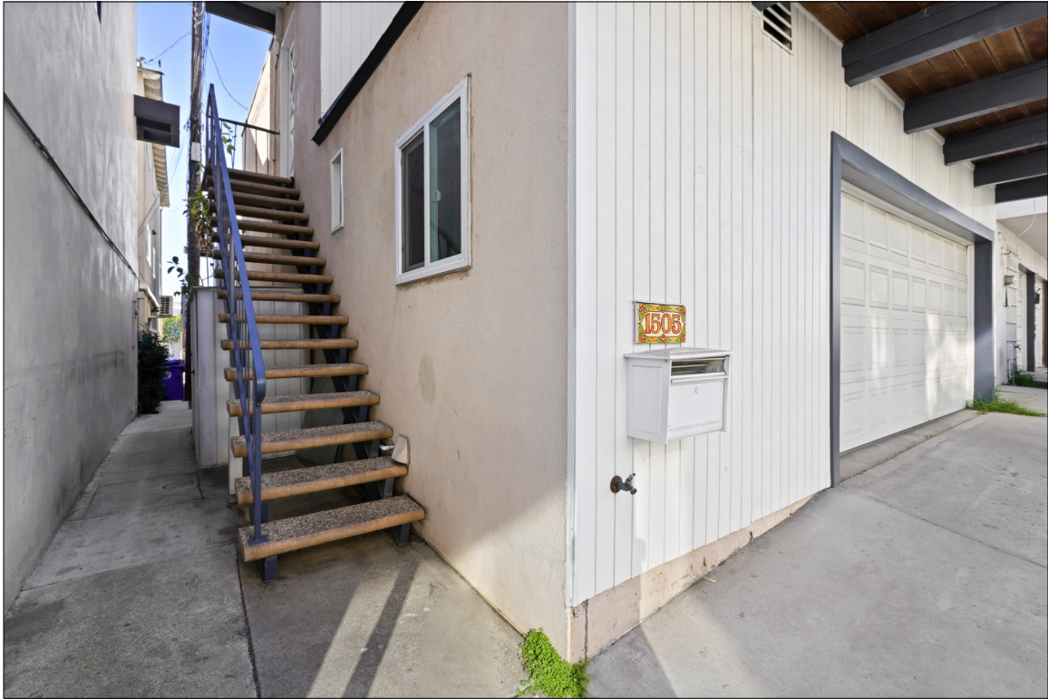
Photo 3: 1505 Crest Drive, south elevation, view northwest (source: Snow, 2021)
