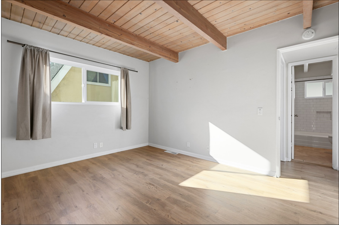
Photo 11: 1505 Crest Drive, interior, second floor bedroom, view northwest (source: Zach Kluckxon, 2021)
