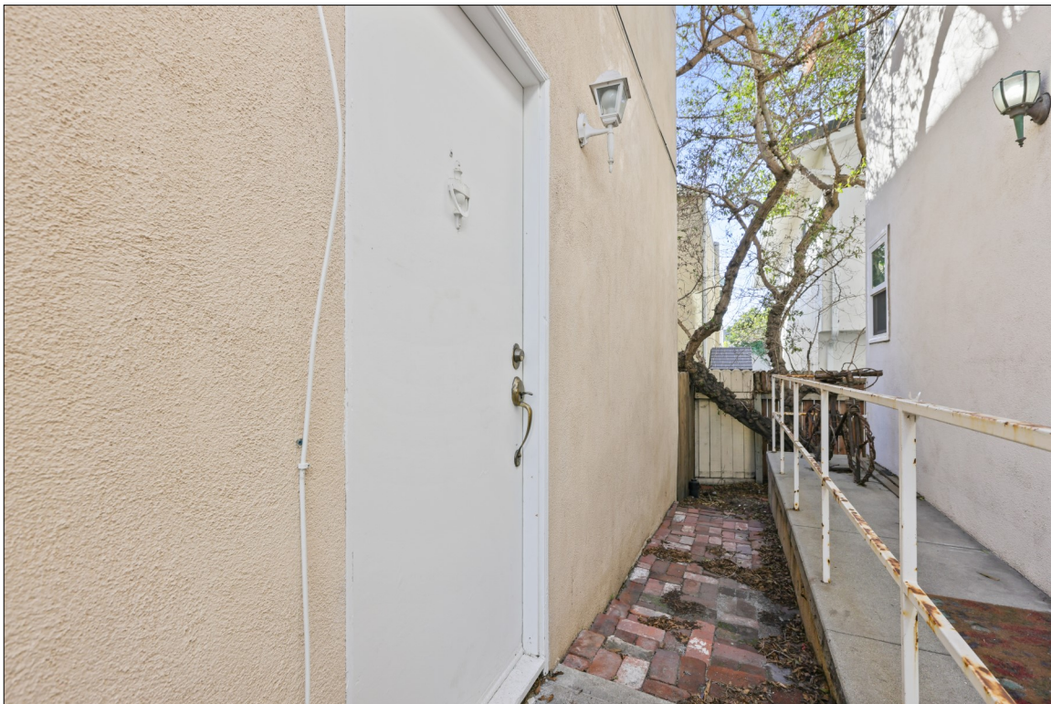
Photo 6: 1505 Crest Drive, north elevation, view southwest, note entrance to rumpus room (source: Snow, 2021)
