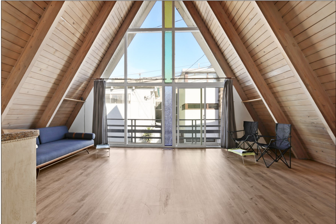
Photo 7: 1505 Crest Drive, interior, living room/dining room, view east toward glazing in gable end (source: Zach Kluckxon, 2021)
