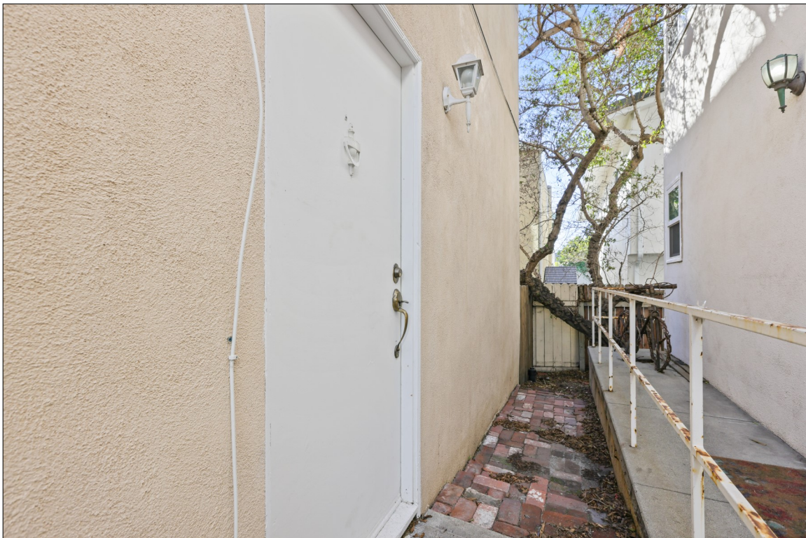
Photo 6: 1505 Crest Drive, north elevation, view southwest, note entrance to rumpus room (source: Snow, 2021)
