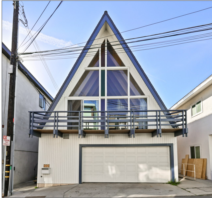
Photo 1: 1505 Crest Drive, east elevation, view west (source: Zach Kluckxon, 2020)
