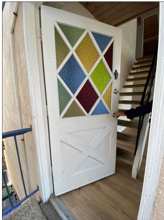
Photo 4: 1505 Crest Drive, primary entrance at second floor, view northwest (source: Snow, 2021)
