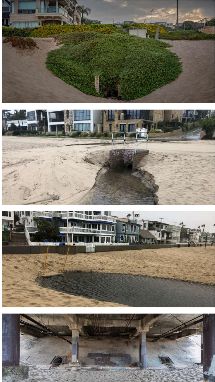
Figure 3-8. Stormwater Outfalls onto the Beach that Drain Higher Areas of the City
