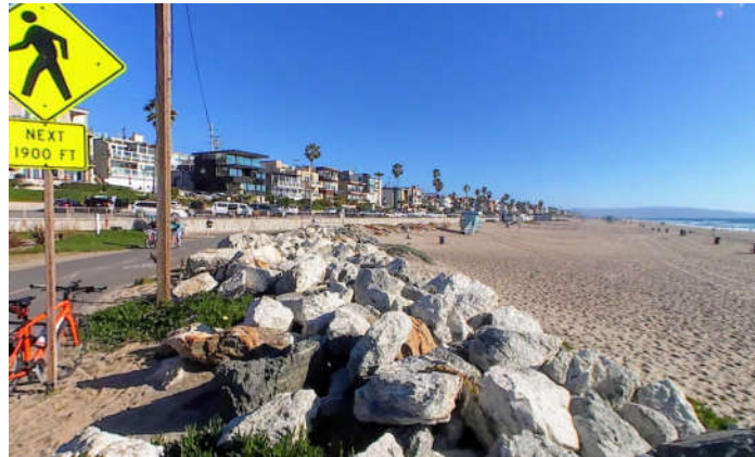
Figure I-4. Existing Rock Revetment at North End of El Porto Beach
