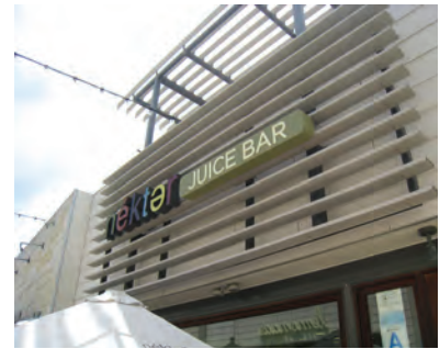
Figures 26 - 27 Signage should be high-quality, pedestrian-oriented, and compatible with the building style
