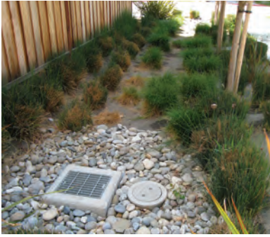
Figure 25 Vegetated bioswale filters stormwater
