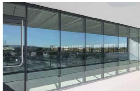
3 Curtain Wall Glazing
