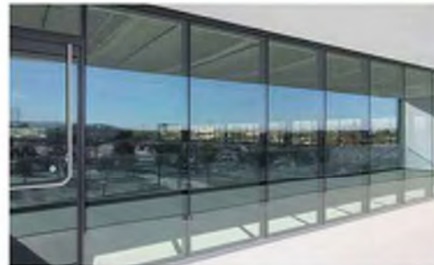
3 Curtain Wall Glazing
