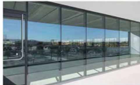
3 Curtain Wall Glazing
