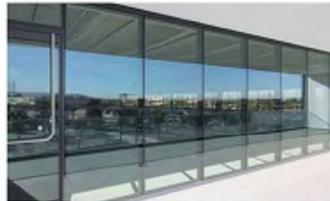
3 Curtain Wall Glazing
