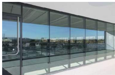
3 Curtain Wall Glazing
