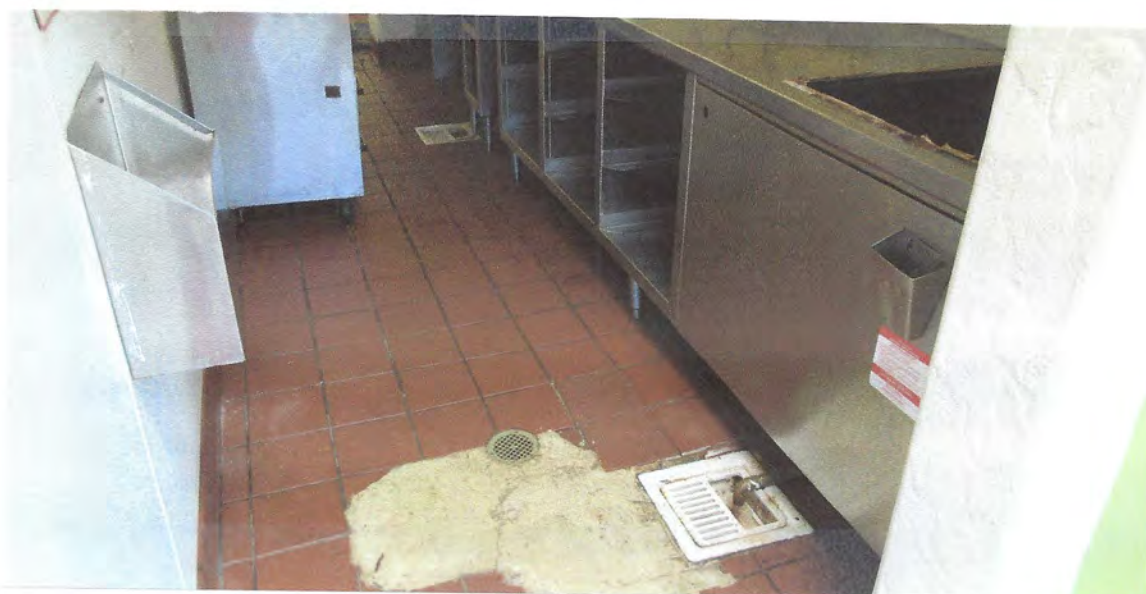
Photographs 8, 9 and 10 - Views of an electrical transformer near the southeast corner of the site building; and views of the vacant kitchen area of the building.
