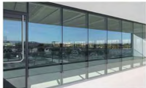
3 Curtain Wall Glazing
