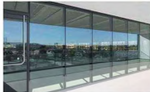
3 Curtain Wall Glazing
