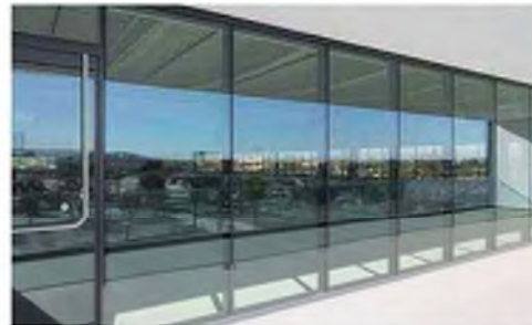
3 Curtain Wall Glazing
