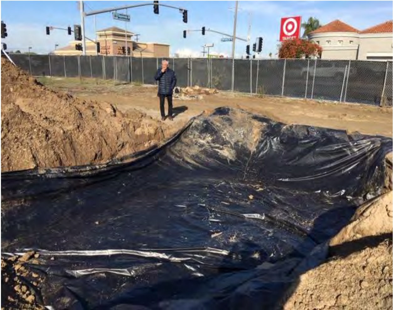
Photo 5: Placement of 6 mil plastic liner at 5 ft bgs
