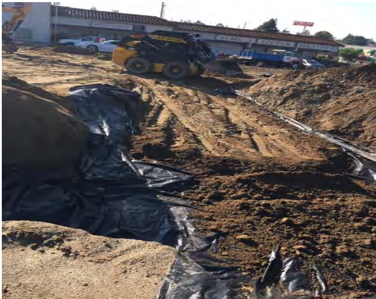
Photo 6: Backfilling of top of excavated area
