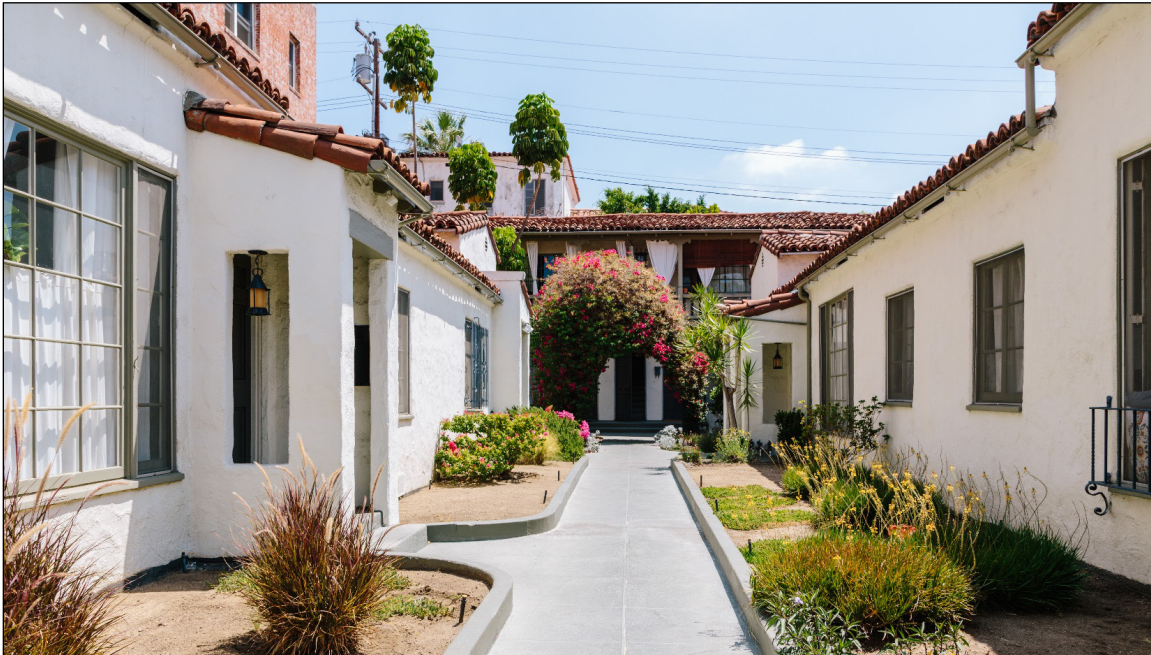
Figure 7: 1230-32 Flores Street, 2015. This building is a designated example of the Spanish Colonial Revival style in West Hollywood. It is listed locally as a contributor to the Courtyard Thematic District (Tony Coelho, City of West Hollywood).
