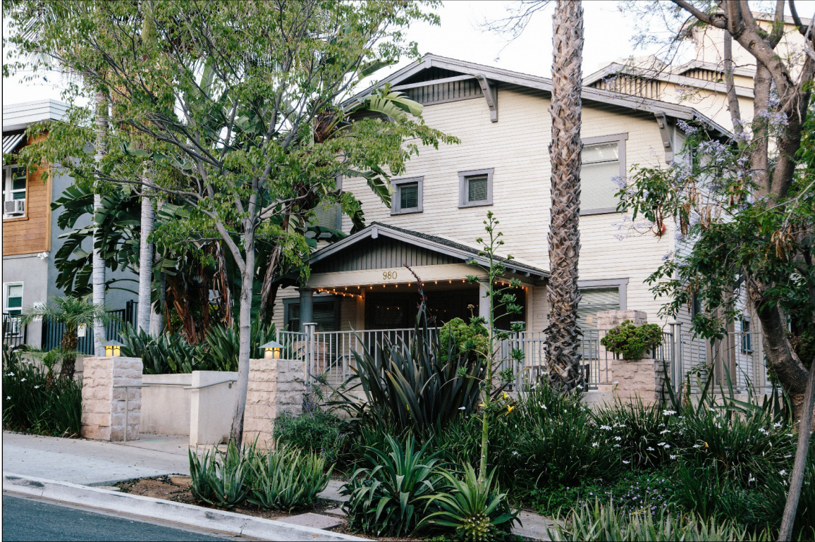
Figure 5: 980 Palm Avenue, 2020. This multi-family building is a designated example of the Craftsman style in the City of West Hollywood. It is listed locally as a contributor to the West Hollywood Craftsman Thematic District (Tony Coelho, City of West Hollywood).
