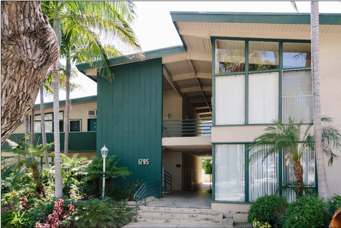
Figure 16: The Fountain Lanai (1285 Sweetzer Avenue), 2015. This building is a designated example of the Mid-Century Modern style that is individually listed as a West Hollywood Cultural Resource (Tony Coelho, City of West Hollywood).
