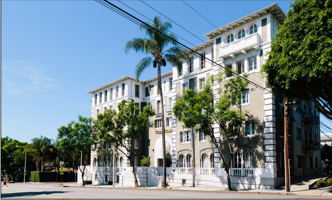
Figure 8: Villa Italia (1201 Crescent Heights Boulevard), 2015. This building is a designated example of the Mediterranean Revival style that is individually listed as a West Hollywood Cultural Resource (Tony Coelho, City of West Hollywood).
