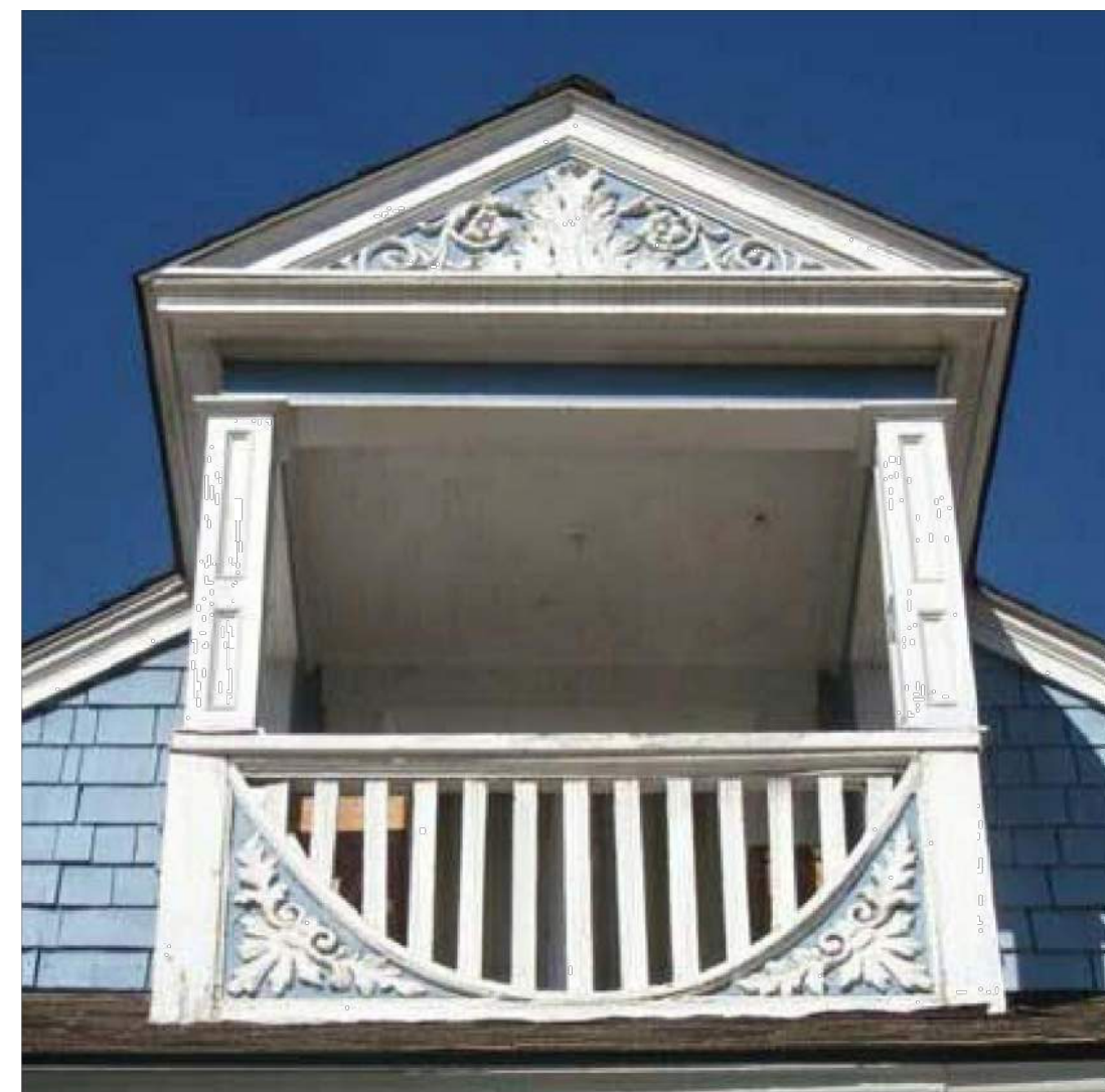
IMAGE: 850 SAN VICENTE. SAMPLE IMAGE OF BALCONETTE AND DETAILING TO BE RETAINED
