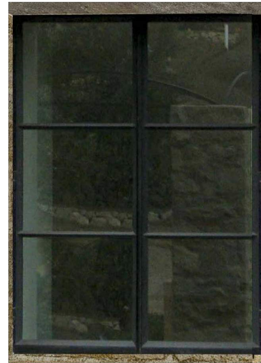
IMAGE: STEEL/ALUMINUM WINDOWS. PAINTED STEEL TO BE USED ON NEW CONSTRUCTION AT WEST PROPERTY WITH PUBLIC USE FUNCTIONS. KYNAR PAINTED ALUMINUM TO BE USED ON EAST PROPERTY NEW CONSTRUCTION.
