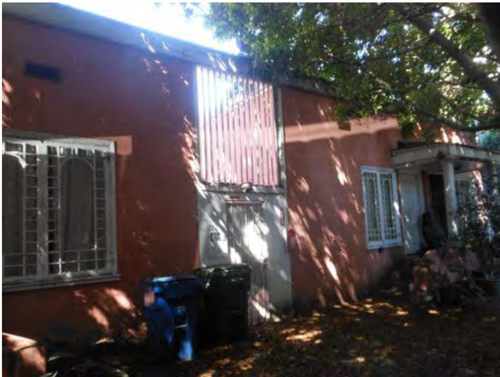
68. Center bay of south (side) elevation looking east
