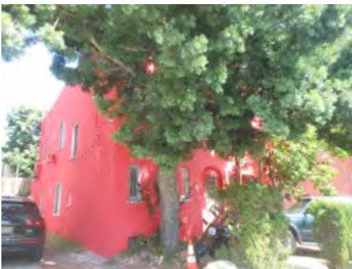
North and west (front) elevations
