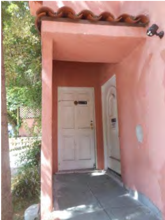
58. Lower level of entry portico
