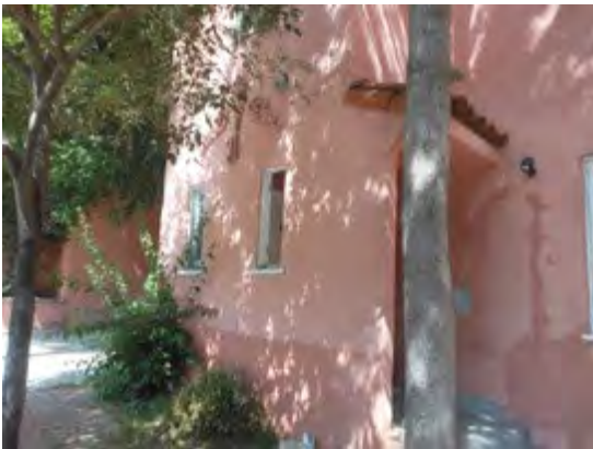
Wing and entry portico on west elevation
