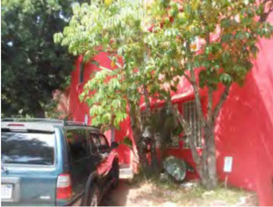
Lower-level west (front) elevation
