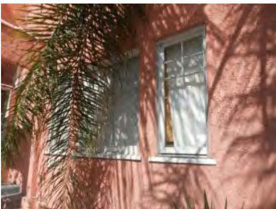
Lower-level west (front) elevation
