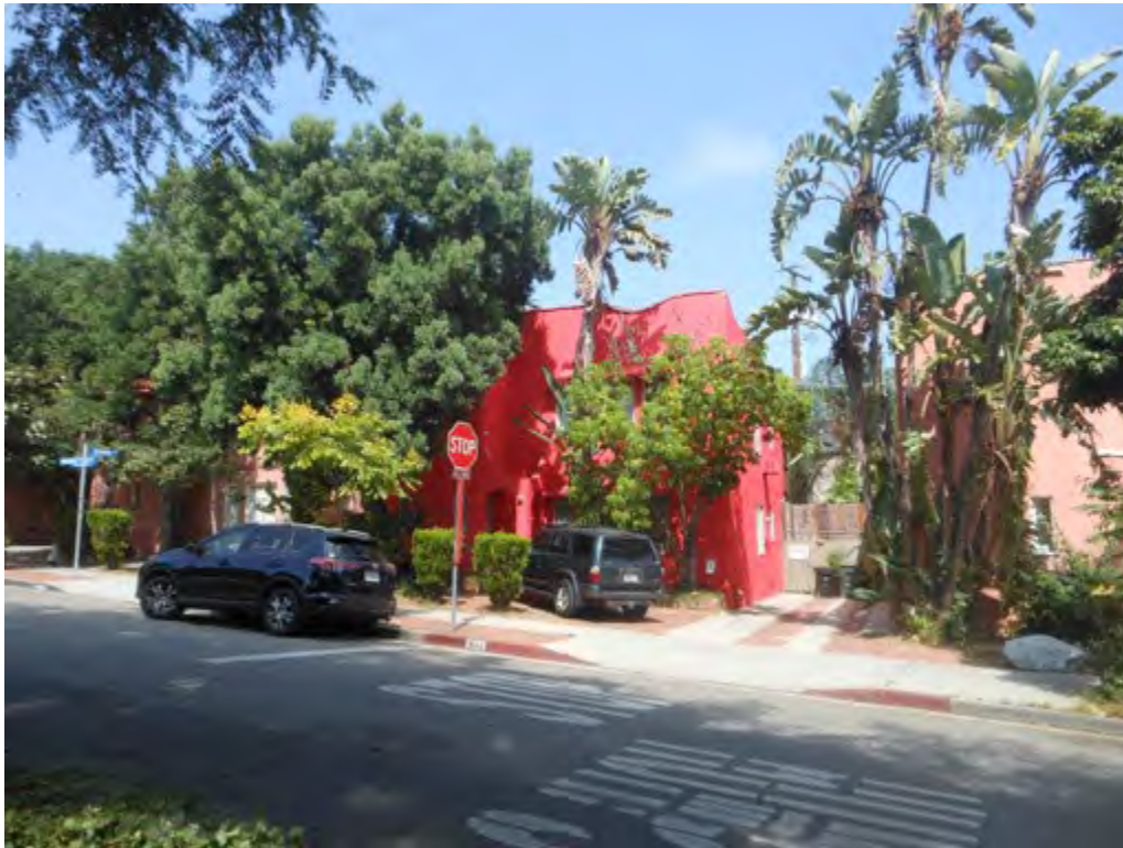
39. West (front) and south elevations
