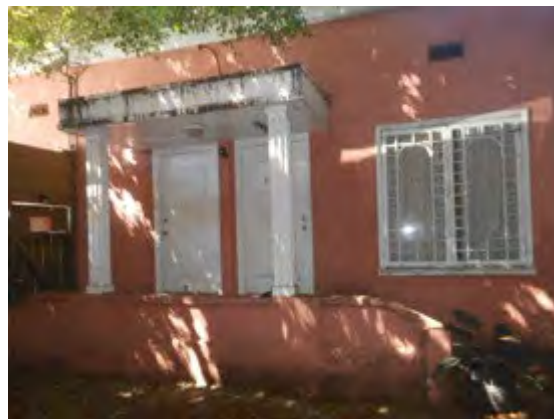
Doorways at porch at west end of south (side) elevations
