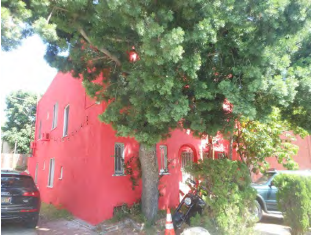
41. North and portion of west (front) elevations
