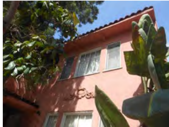
Upper level of west (front) elevation
