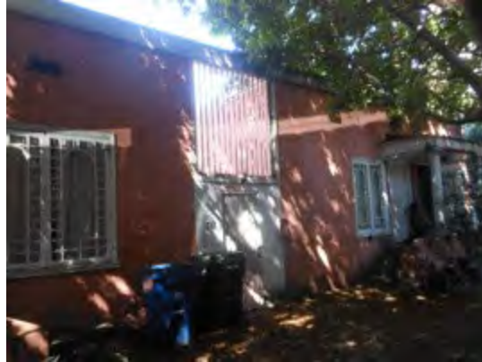
Center bay of south (side) elevation looking east
