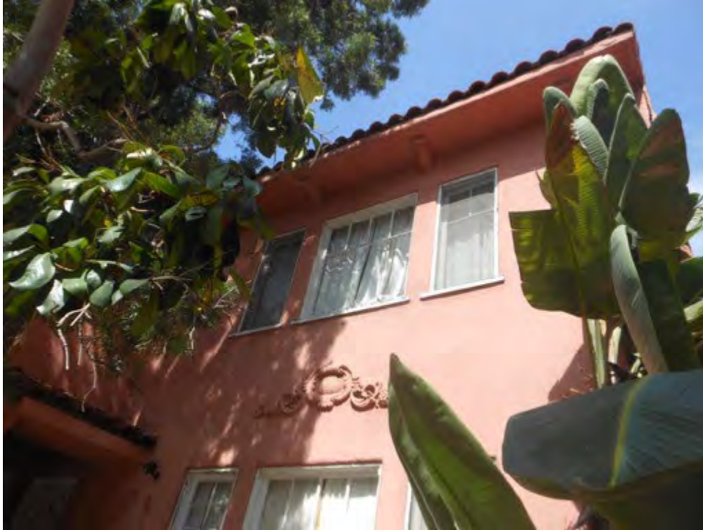
55. Upper portion of west (front) elevation
