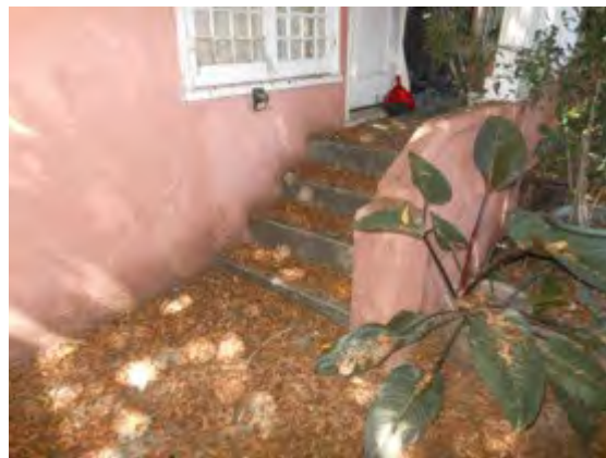
Stairs to porch landing
