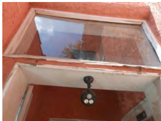
Window above entry portico
