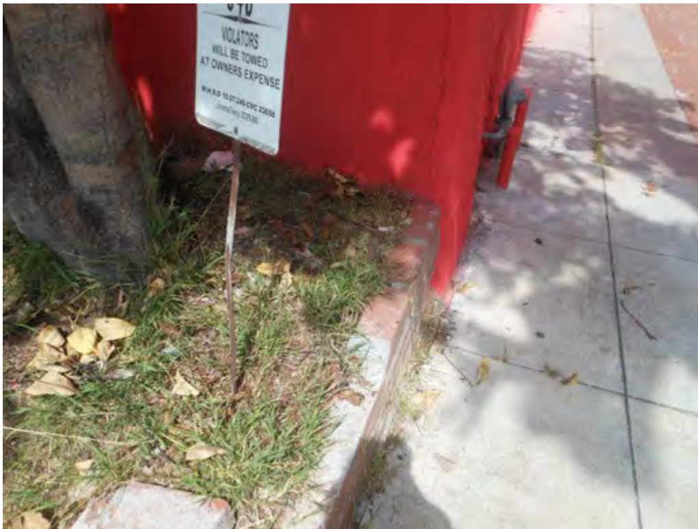
46. Brick planter and paving at south end of west (front) elevation
