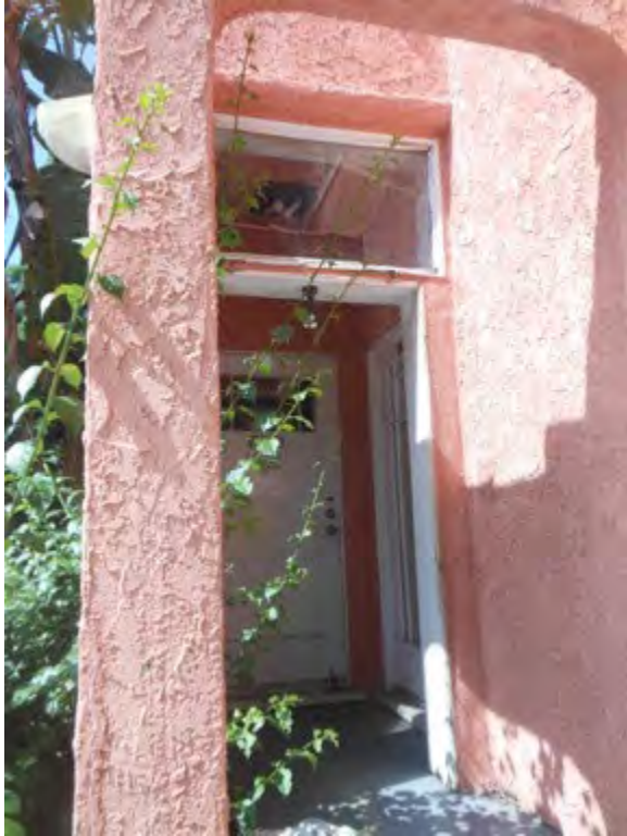
31. Doorway in entrance portico
