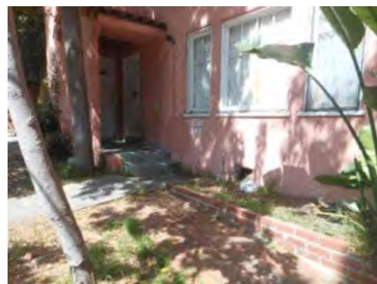
Entry portico and windows on west elevation
