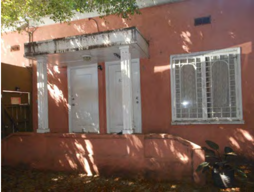
71. Doorways at porch at west end of south (side) elevation
