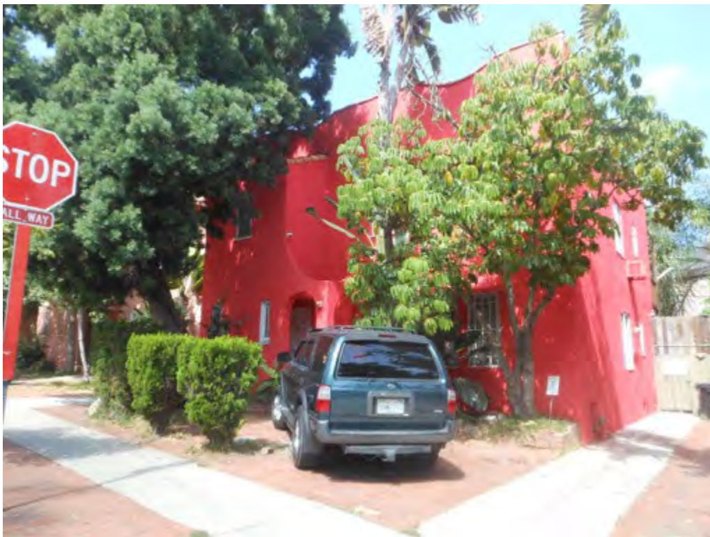
40. West (front) and south elevations
