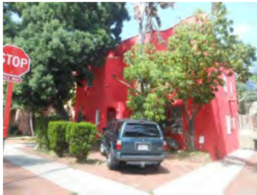
West (front) and south elevations
