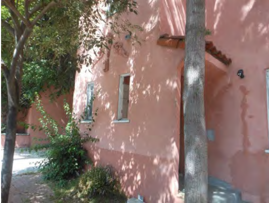
53. Entrance portico on west (front) elevation
