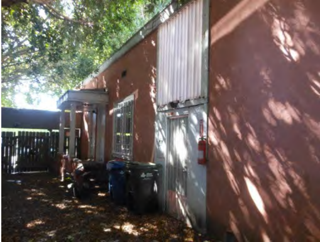
69 Center bay of south (side) elevation looking west
