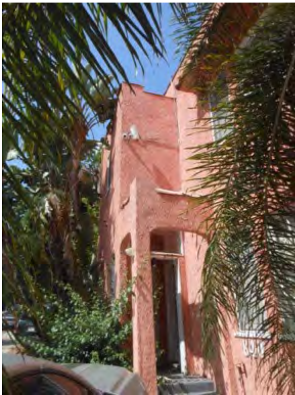
30. Entrance portico on west (front) elevation
