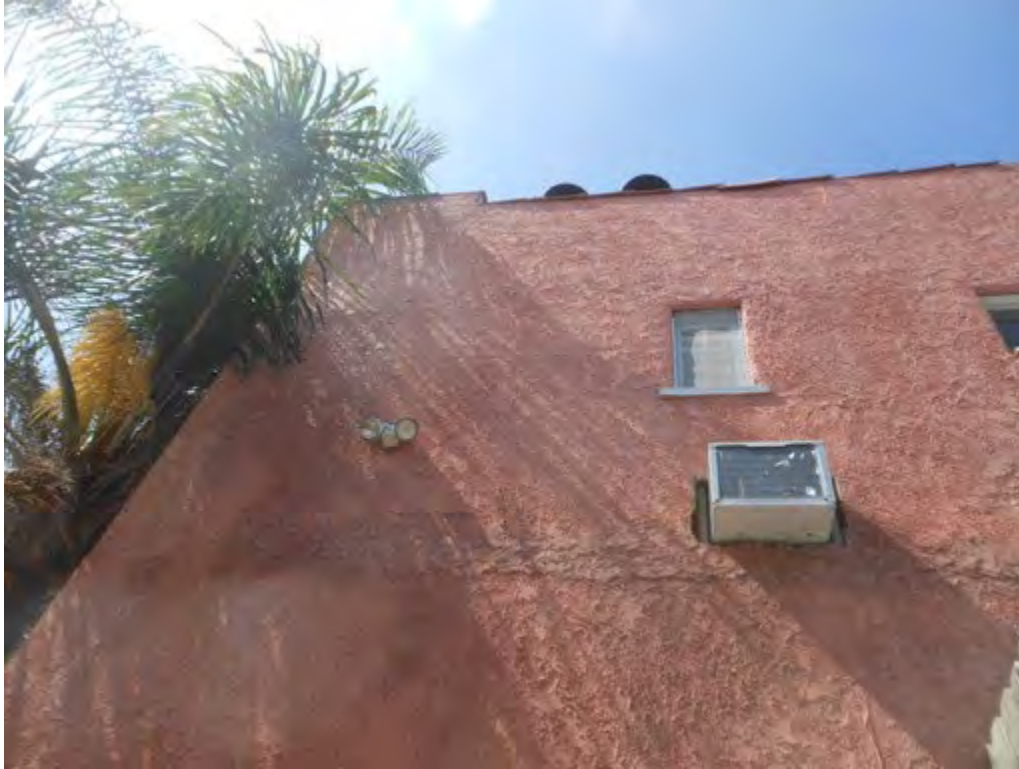
37. Upper level of south elevation
