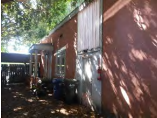
Center bay of south (side) elevation looking west
