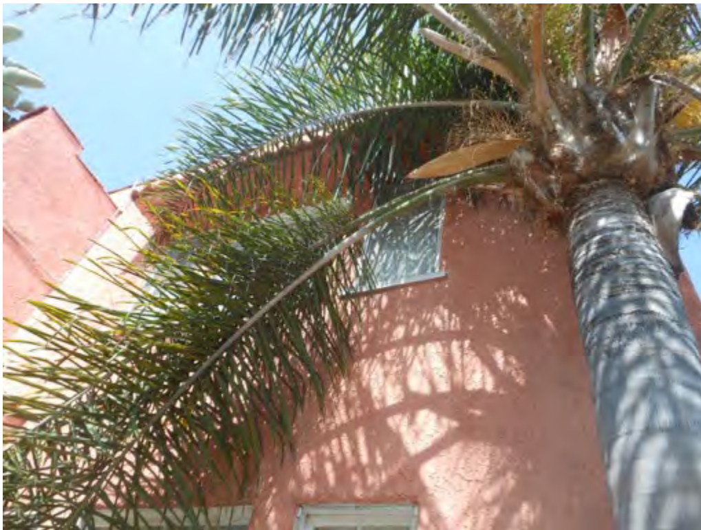
28. Upper level of west (front) elevation
