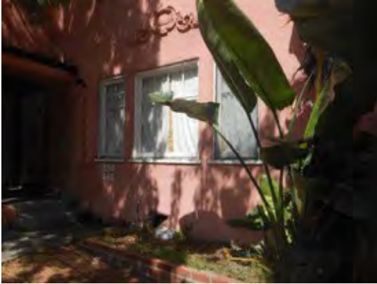
Lower-level windows on west elevation
