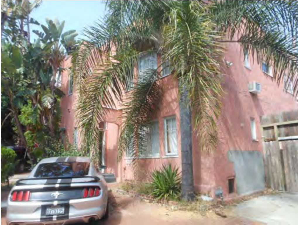
27. West (front) and south elevations
