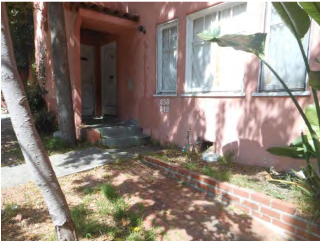
56. Lower portion of west (front) elevation
