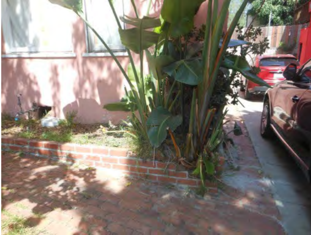
59. Planter along west (front) elevation
