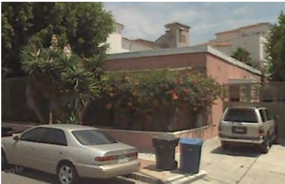
66. West (front) and south elevations at driveway in 2007 (Google Maps)
