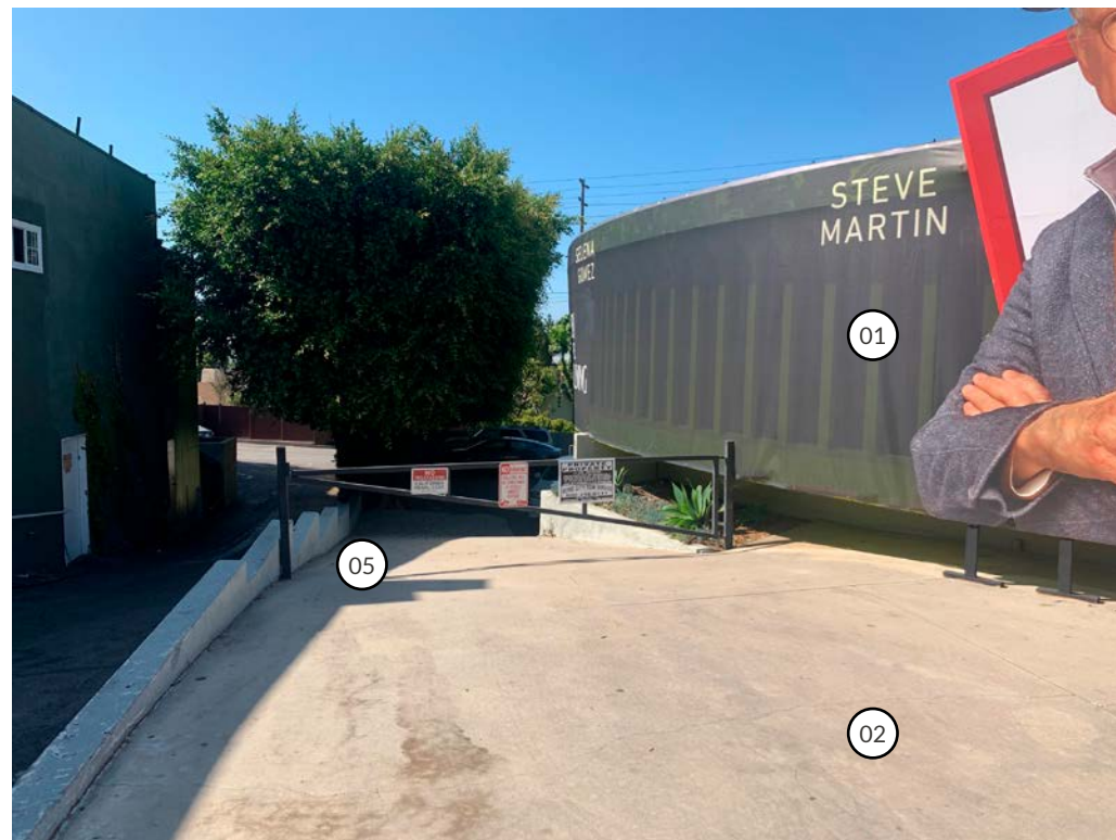
Front View of NW Corner of Building
