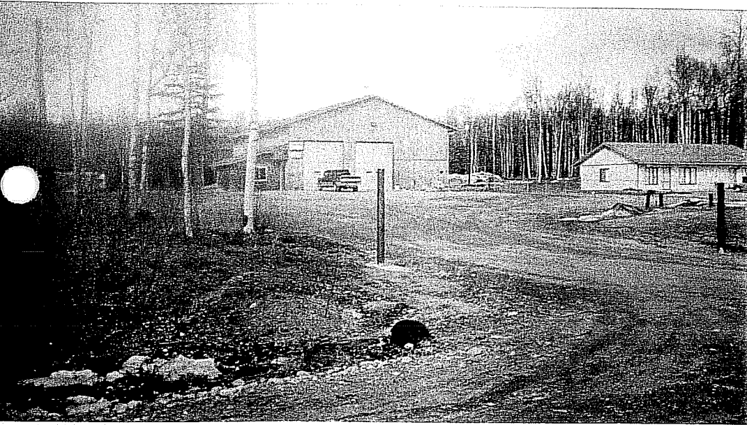
View North Shop/Warehouse
