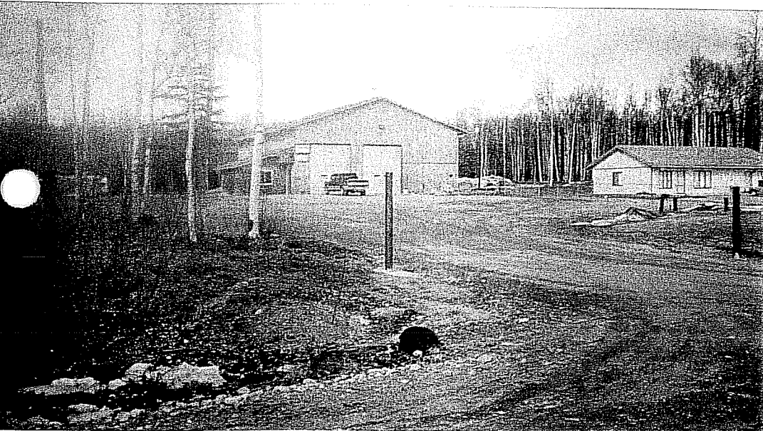
View North Shop/Warehouse
