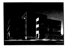
The lower floor of the building is finished with an exterior insulation and finish system, while the upper floors are clad in insulated metal panels. The facility's interior incorporates 10' 6" ceilings and light shelves at the windows, which bounce natural light deep into the building's interior. The interior fixtures and finishes were carefully selected to enhance the work environment while maintaining the professional image desired by Alyeska.
