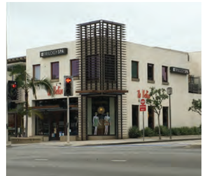
Figure 2 Corner entrance emphasized through unique articulation and materials
