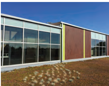
Figure 36 Green roofs absorb heat and rainwater
