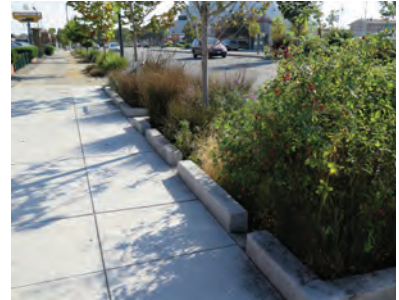
Figures 37 - 38 Planting strips and bioswales help reduce and filter stormwater
