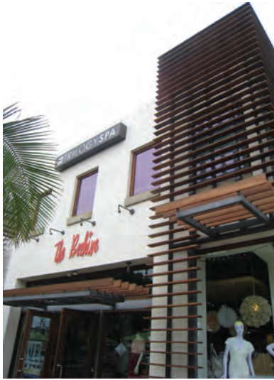
Figure 12 Awnings provide cover for pedestrians
