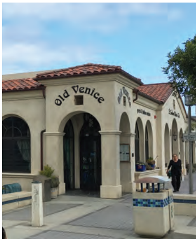
Figure 4 Inviting corner entrance with tower feature
