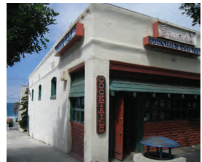
Figure 17 1101 Manhattan Ave is the oldest commercial building in the Downtown
