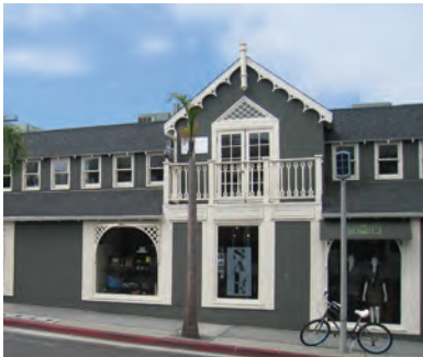
Figure 8 Detailed architectural treatments enhance the facade
