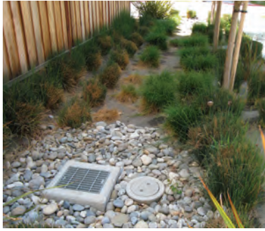
Figure 25 Vegetated bioswale filters stormwater
