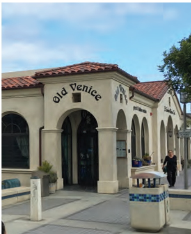
Figure 4 Inviting corner entrance with tower feature
