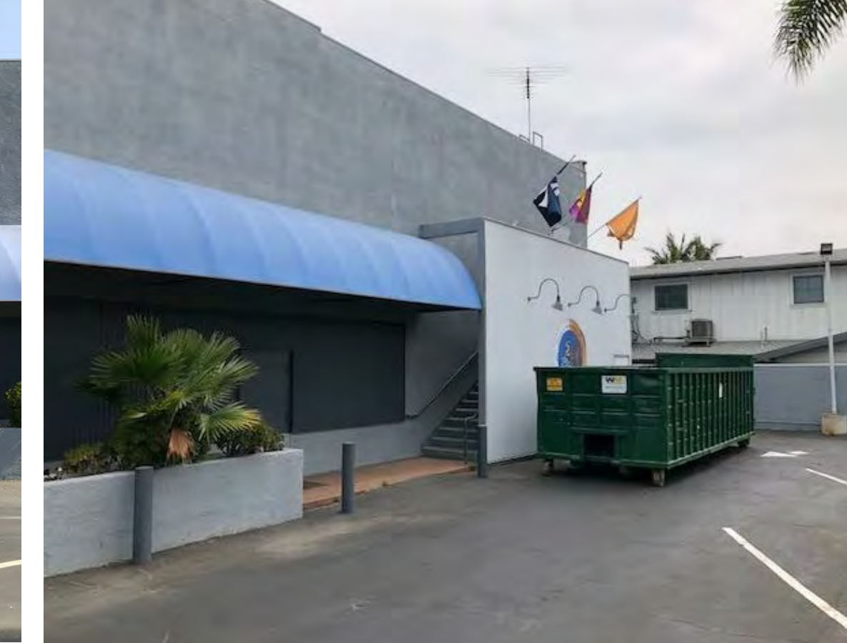
CURRENT SOUTH FACADE
