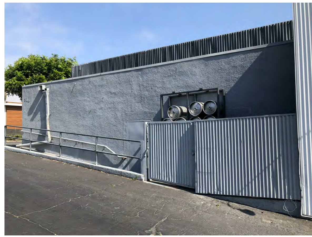
CURRENT SOUTH FACADE
