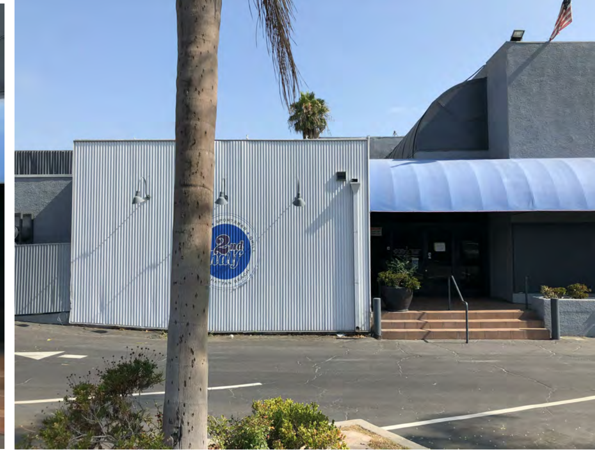
CURRENT SOUTH FACADE
