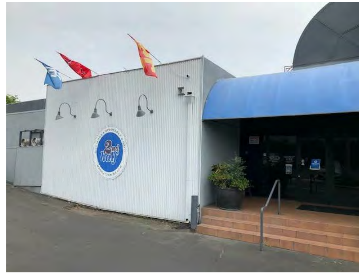
CURRENT SOUTH FACADE
