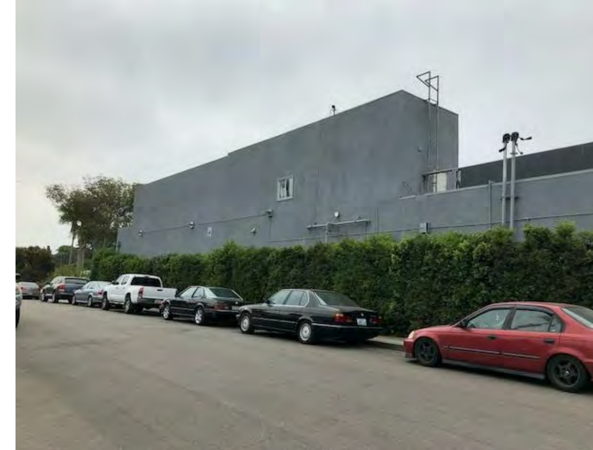
CURRENT NORTH FACADE
