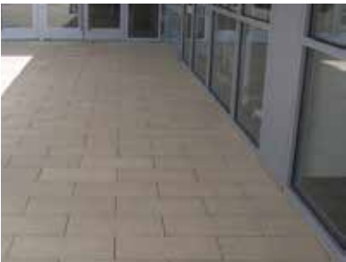
Figures 2-37 Walkways with interlocking pavers
