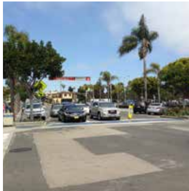
+T3 Yield to pedestrians along Manhattan Beach Boulevard and Morningside is potentially an issue for safety and should be replaced with a controlled intersection.
