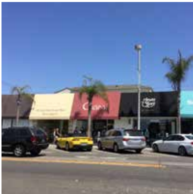
+C3 Angled parking is efficient since it combines backout space with vehicular through movements.
