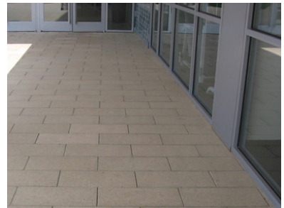
Figures 7.30 Walkways with interlocking pavers
