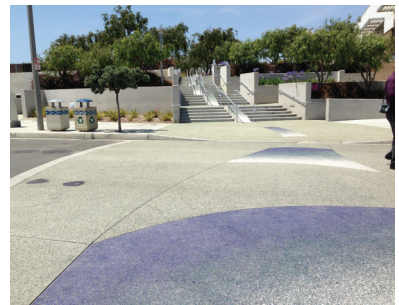
Figures 7.32 Concrete with recycled glass tends to last a long time with few maintenance problems
