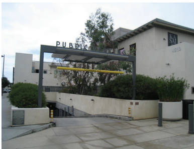
Figure 2.15 Metlox underground parking garage structure
