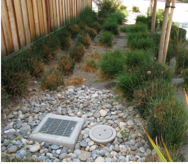
Figure 6.3233 Vegetated bioswale filters stormwater
