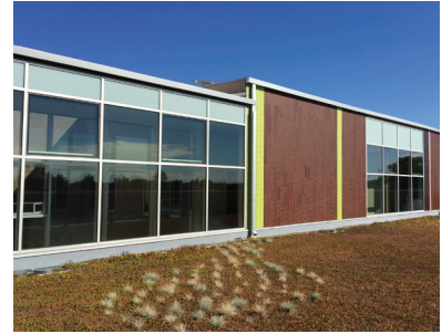
Figure 6.4544 Green roofs absorb heat and rainwater
