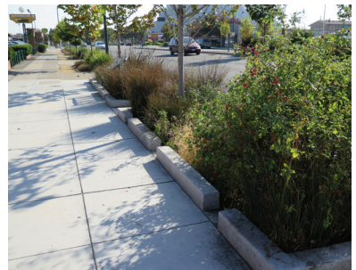
Figures 6.4445-6.4546 Planting strips and bioswales help reduce and filter stormwater
