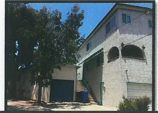
6. Back View (27th Street)
