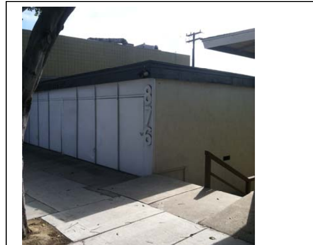
Functionally obsolete building with underutilized capacity.
