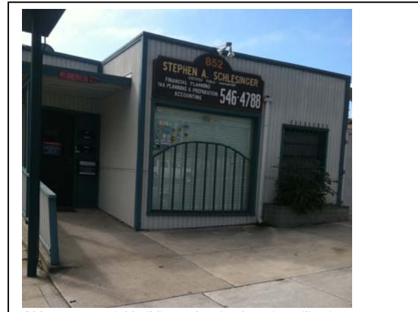
Older commercial buildings showing low site utilization.
