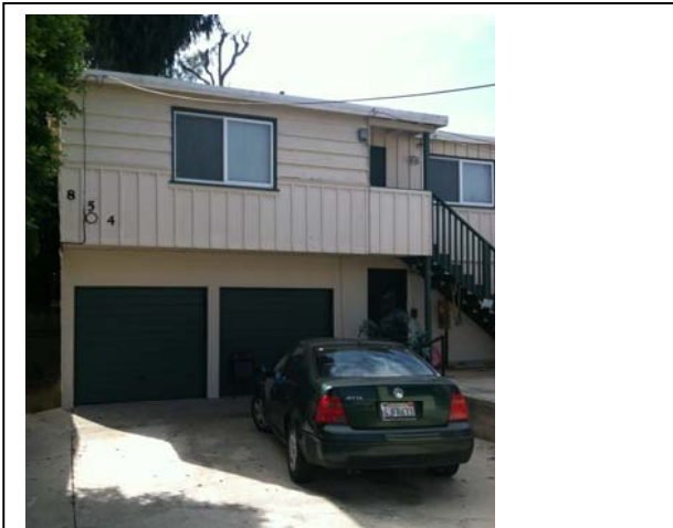
Older, functionally obsolete multi-family building.
