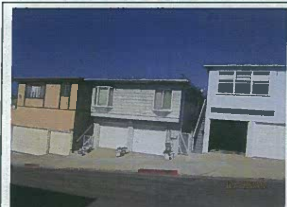
Older, functionally obsolete multi-family buildings showing signs of disrepair.
