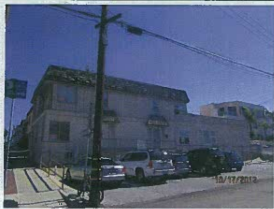
Older underutilized multi-family building showing signs of disrepair and vacancies.
