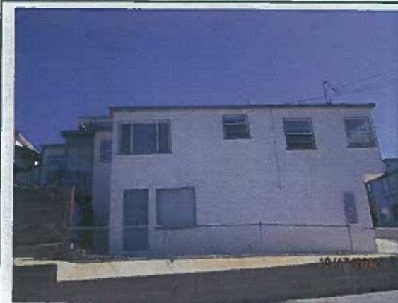
Older underutilized multi-family building showing signs of disrepair and functional obsolescence.
