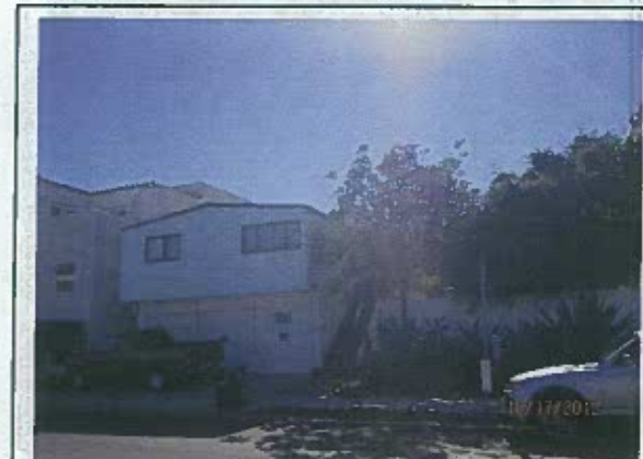
Older multi-family showing deferred maintenance and underutilized capacity.
