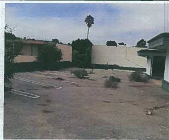
Vacant commercial property with significant deterioration.
