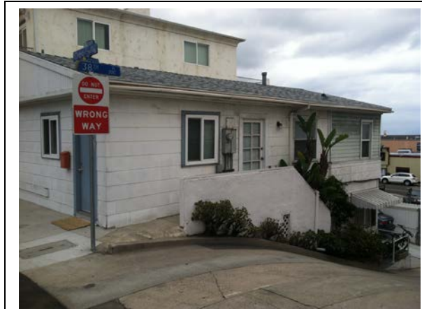
Older multi-family building showing signs of disrepair, low site utilization and functional obsolescence.
