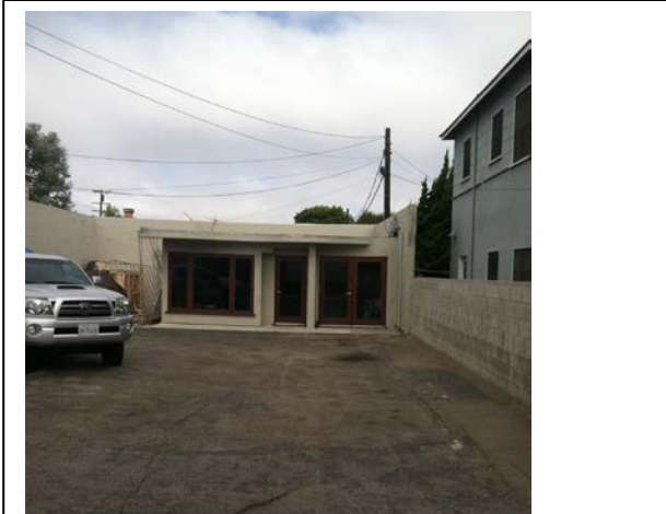
Very low site utilization and disrepair.
