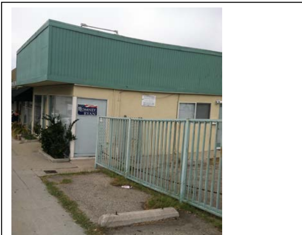
Older single-story commercial building with deferred maintenance and low site utilization.
