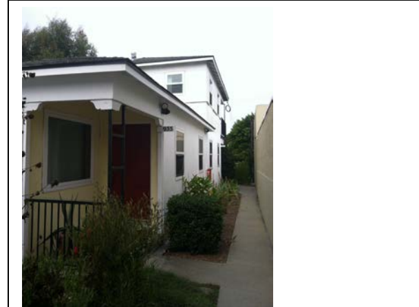
Older multi-family building showing functional obsolescence and low site utilization.
