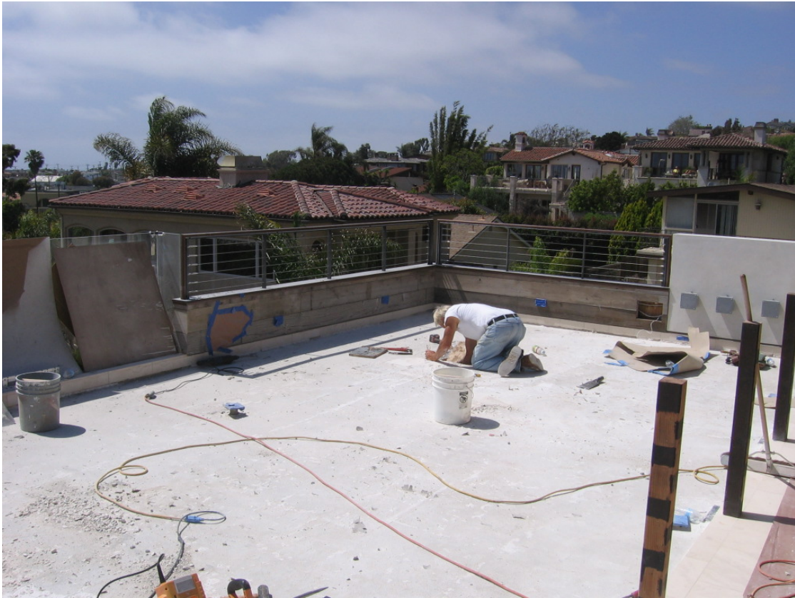
Removal of Tile and Gas Line– Facing Northwest
