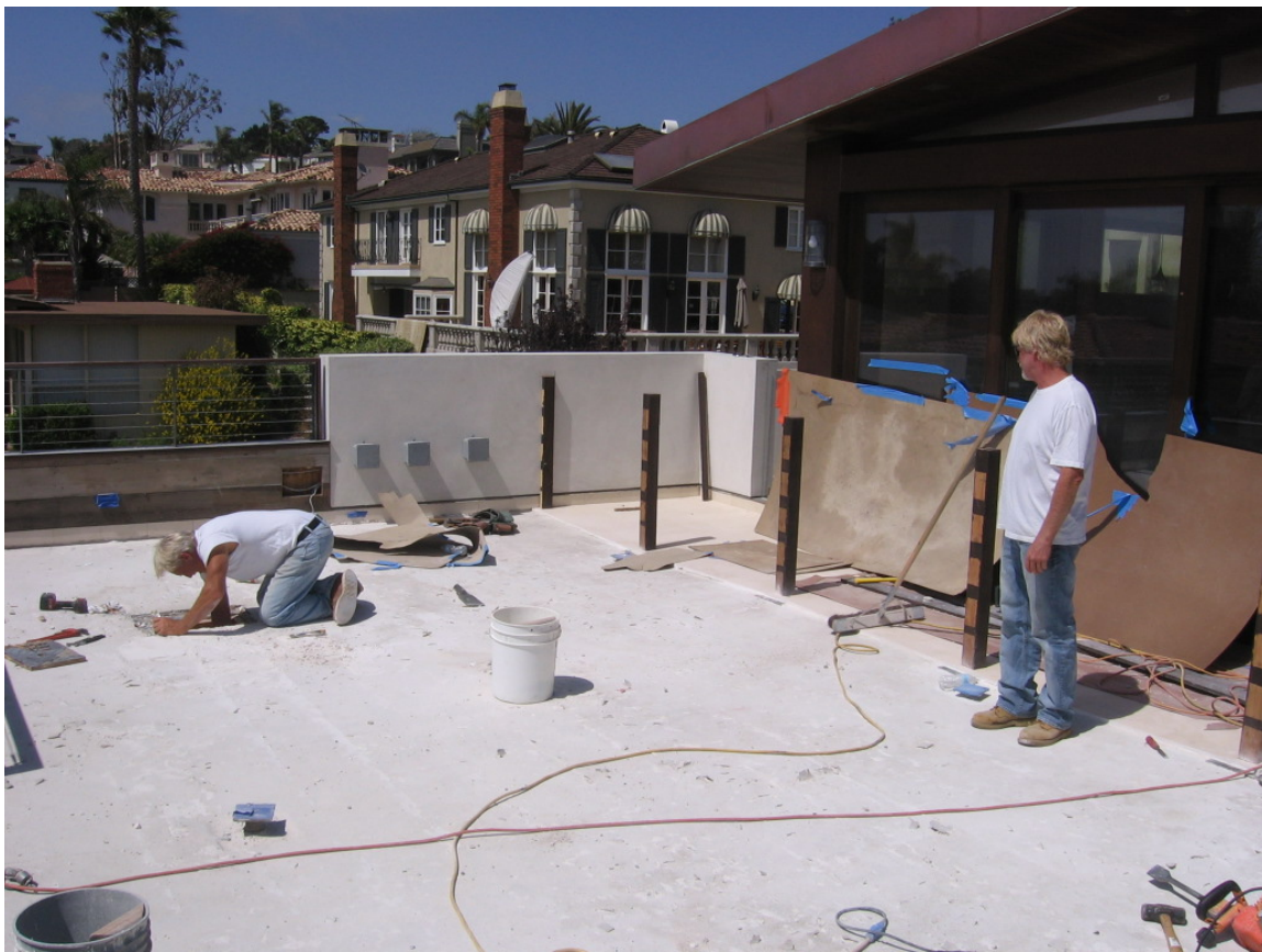
Removal of Tile and Gas Line – Facing North
