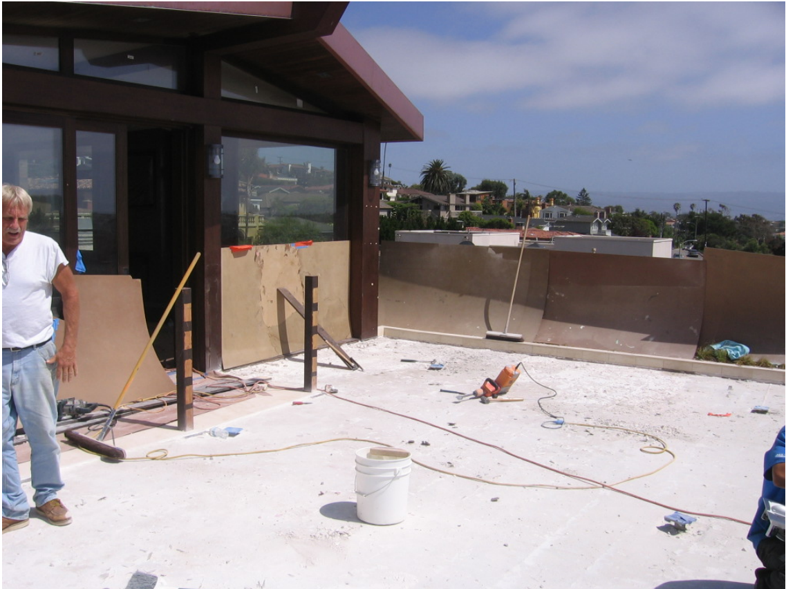
Removal of Tile – Facing South
