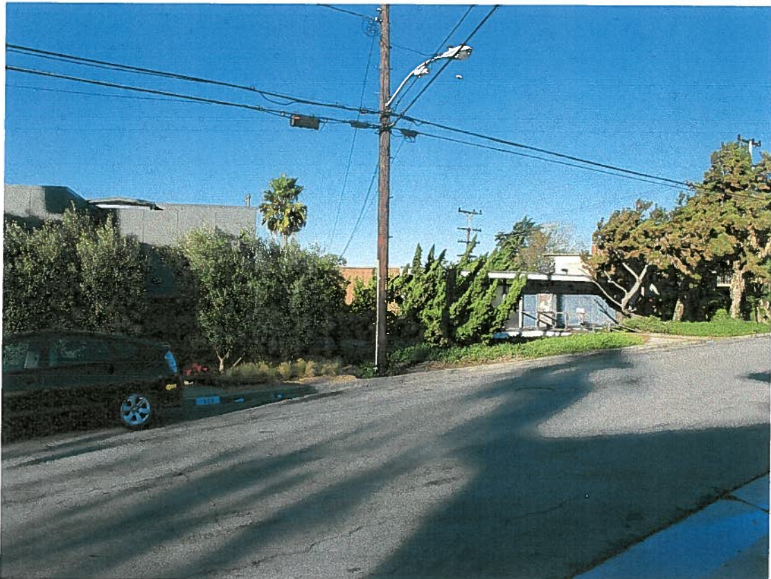
View from Highview Ave. – Existing
