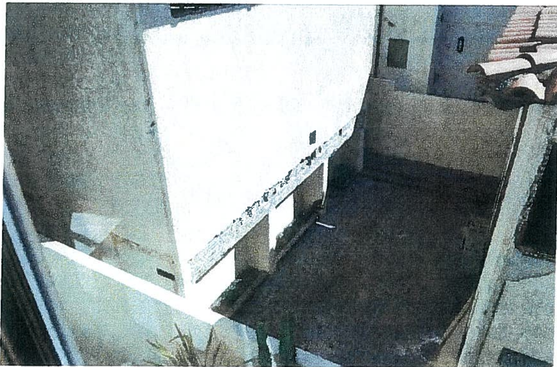
Some of the already removed Stucco
