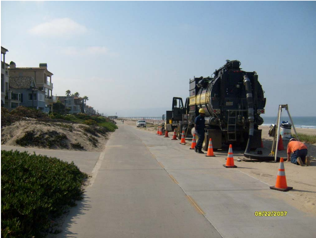
Figure 5 – Unimpeded use of The Strand facilitated by additional concrete pads
