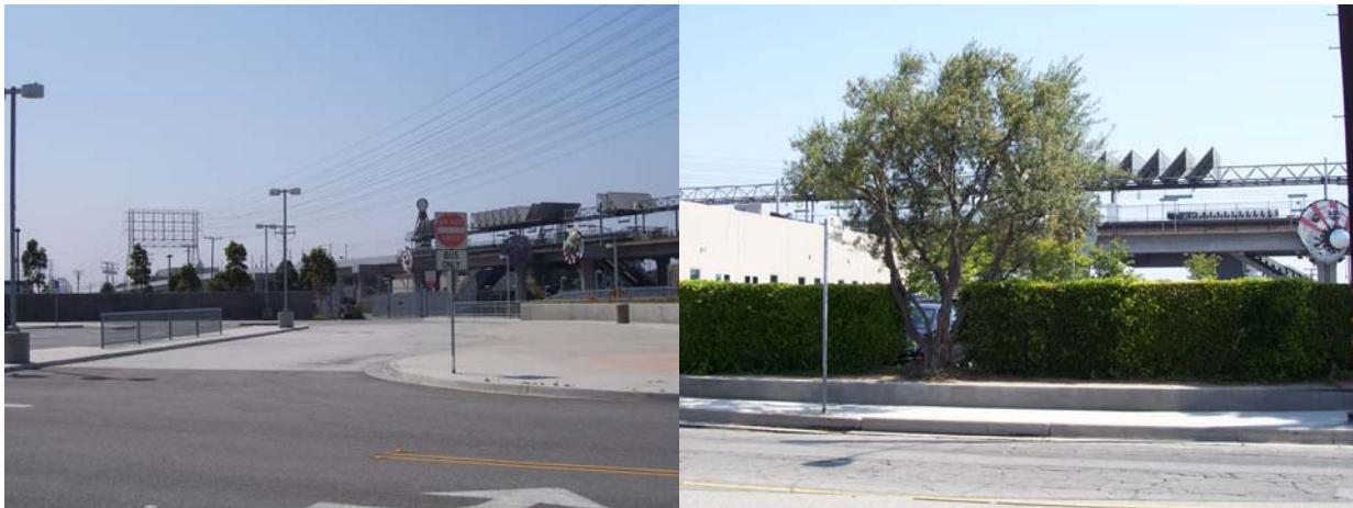
Figure 6.6 BCT Stop at Douglas Station. The photo on the left was the former location; the photo on the right is a view of the station from the current bus stop on Park Place.
