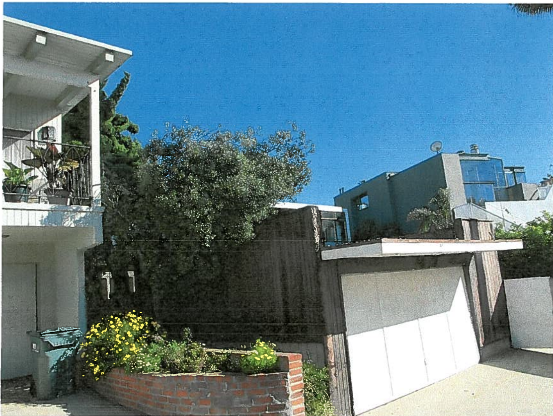
Oblique View from Rear Alley – Existing
