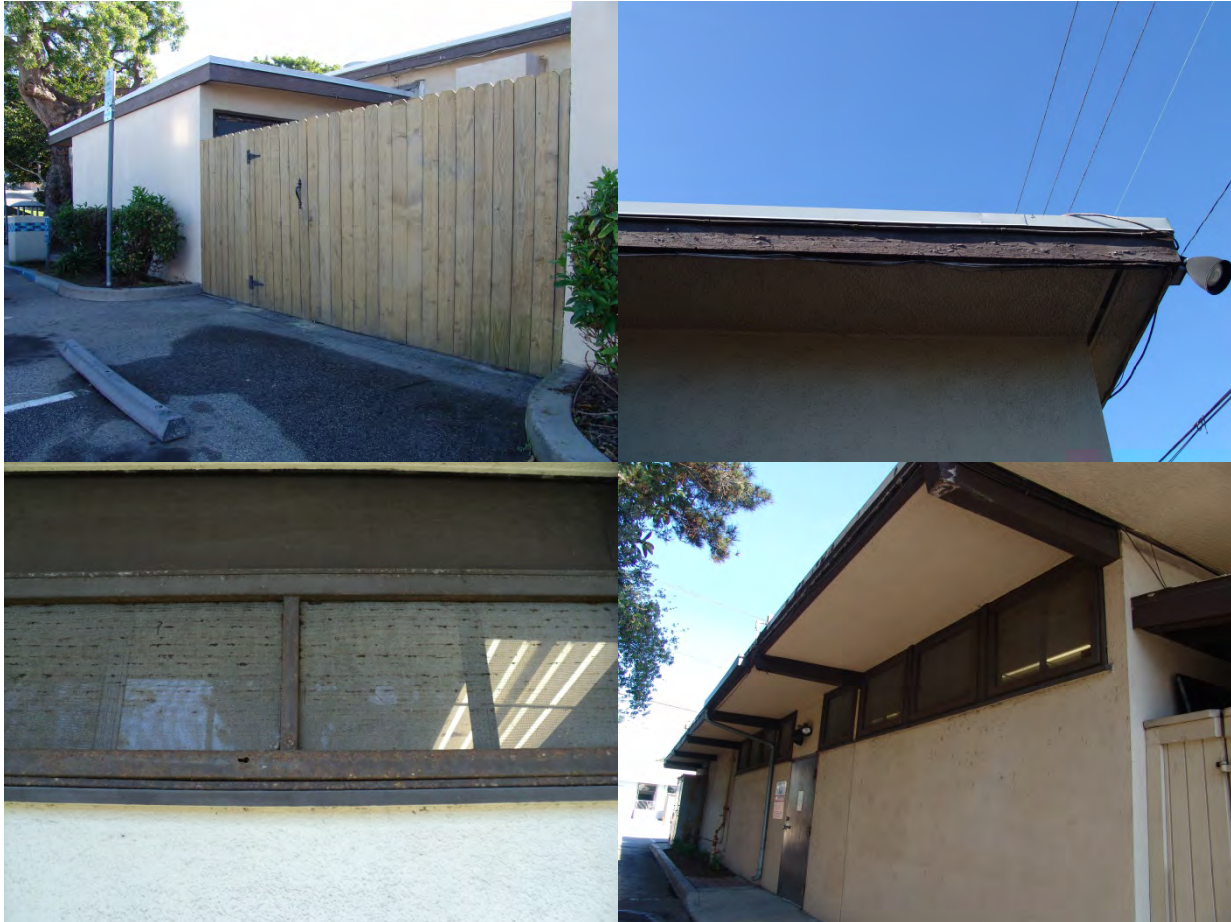
City Hall Annex 425 15 th Street
