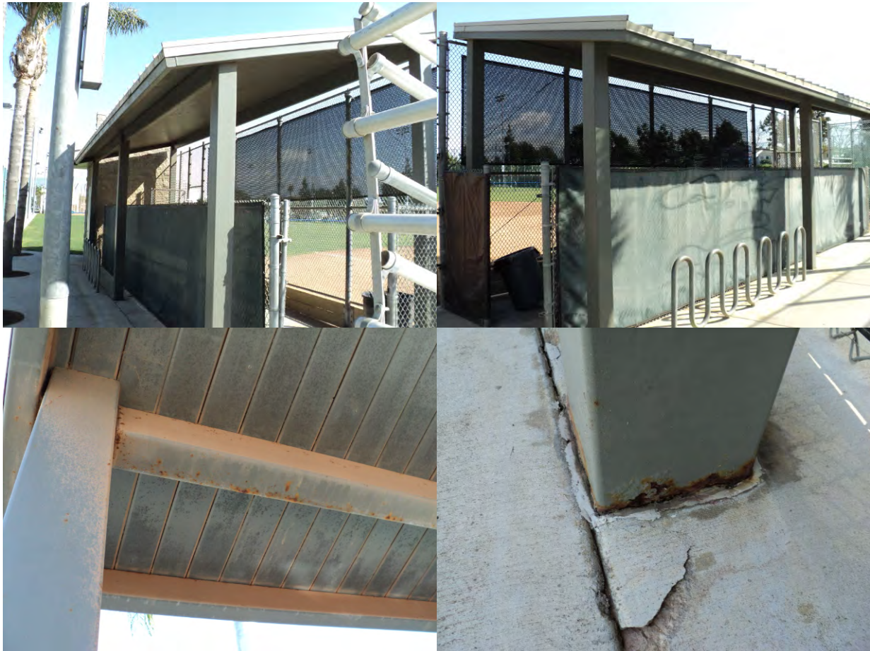
Marine Avenue Sports Complex Dugouts-6 Structures
