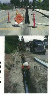
CBM provided design, project management, and construction management for the replacement of aging water pipelines, valves, and water services. Work included replacement of 11,000 LF of 6" and 8" PVC water mains, fire hydrants, valves and fittings, air release/vacuum relief assemblies, flushing risers, and 200 water services. The project was constructed in coordination with the annual street rehabilitation project.
