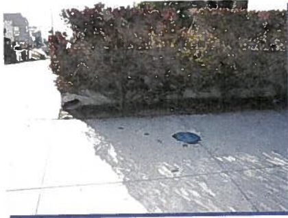
The water valve represents the alignment of the existing water main.
