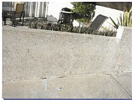
Existing water main location is marked 5 feet inside the private improvements on public right-of-way.
