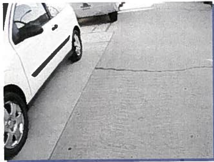
Water main alignment and replaced trench surface pavement.
