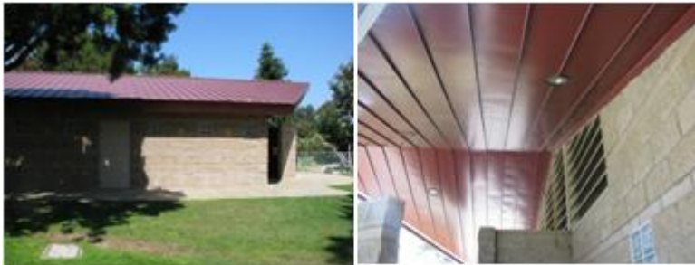
New Restroom Facility
