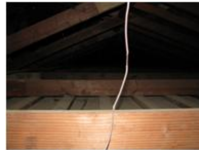
Attic Space in the Scout House
