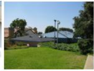
Roof of Chlorine Station and Pumping Station
