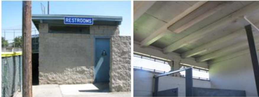
Premier Park Restroom
