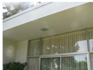
Joslyn Exterior Lighting
