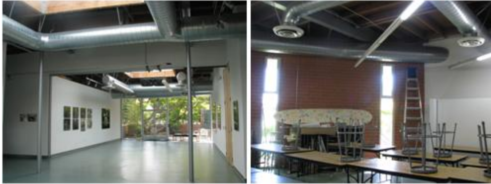
Main Hall with Natural Daylighting
