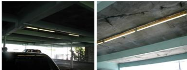
Dark Garage with Rusty Fixtures
