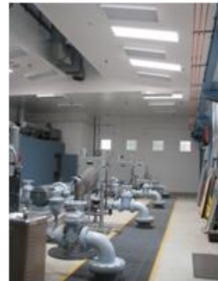
Pumping Station Daylighting
