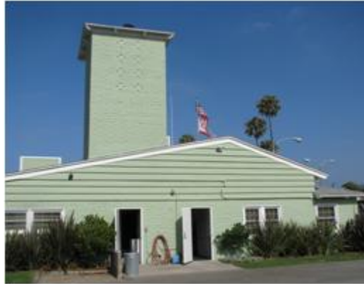
Side view of Fire Station #2
