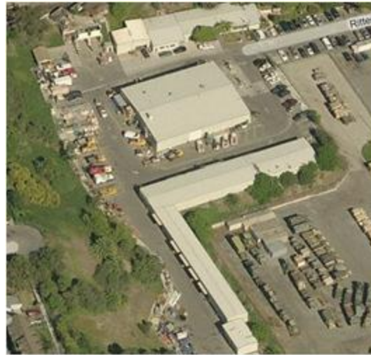
Public Works Yard Photo courtesy of Bing Maps
