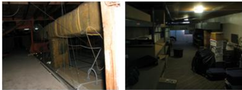
Attic Space in Joslyn C.C.
