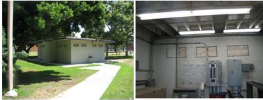
Old Restroom turned into Offices and Storage
