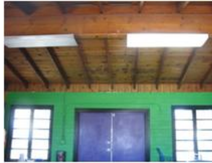
Restroom Bldg/Playground Room
