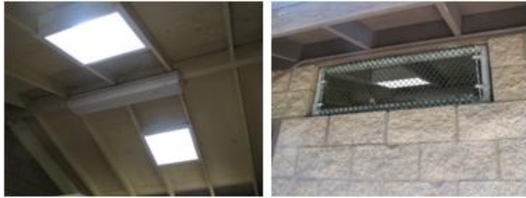
Beach Restroom Daylighting
