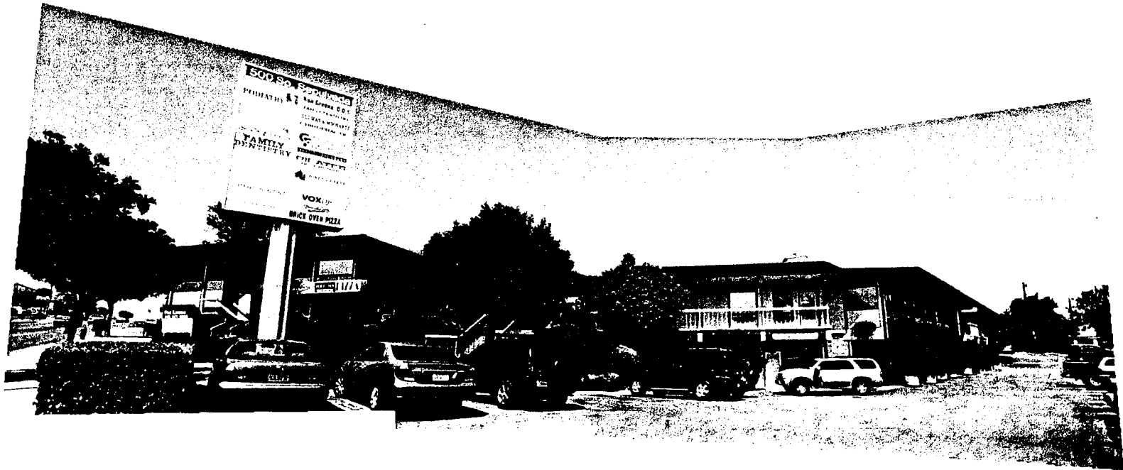
500 S. Sepulveda - Facing towards the Northeast
