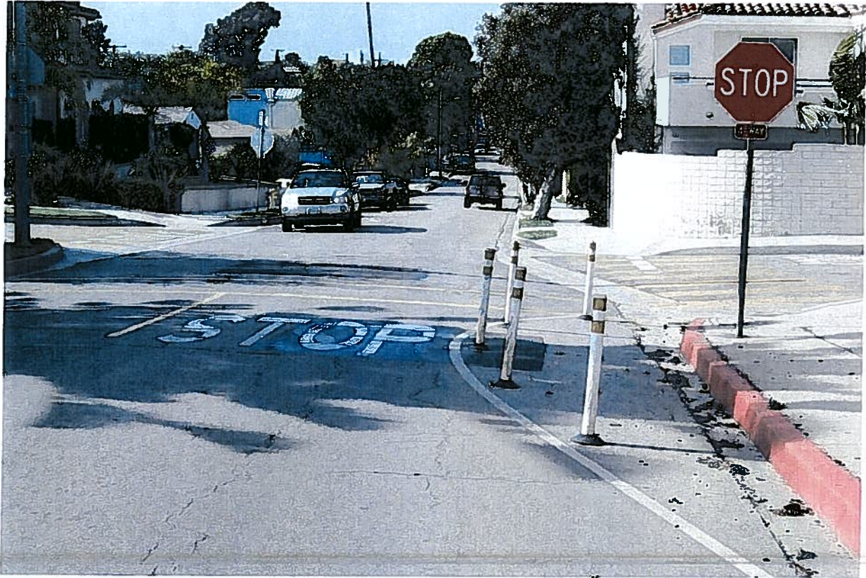
Temporary Bulb-Out at Meadows Ave./17 th Street
