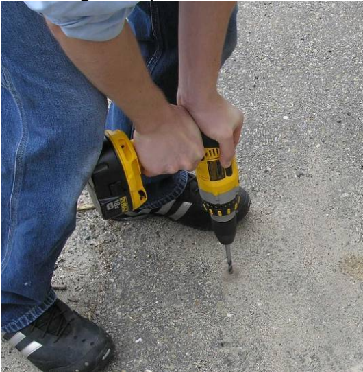
Drilling into pilot holes
