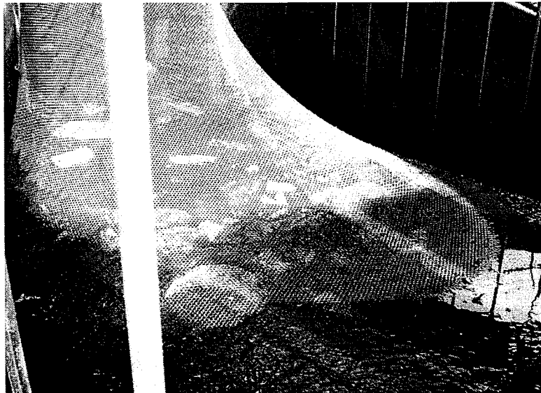
Figure 7 - End-of-pipe net at Hamilton Bowl
