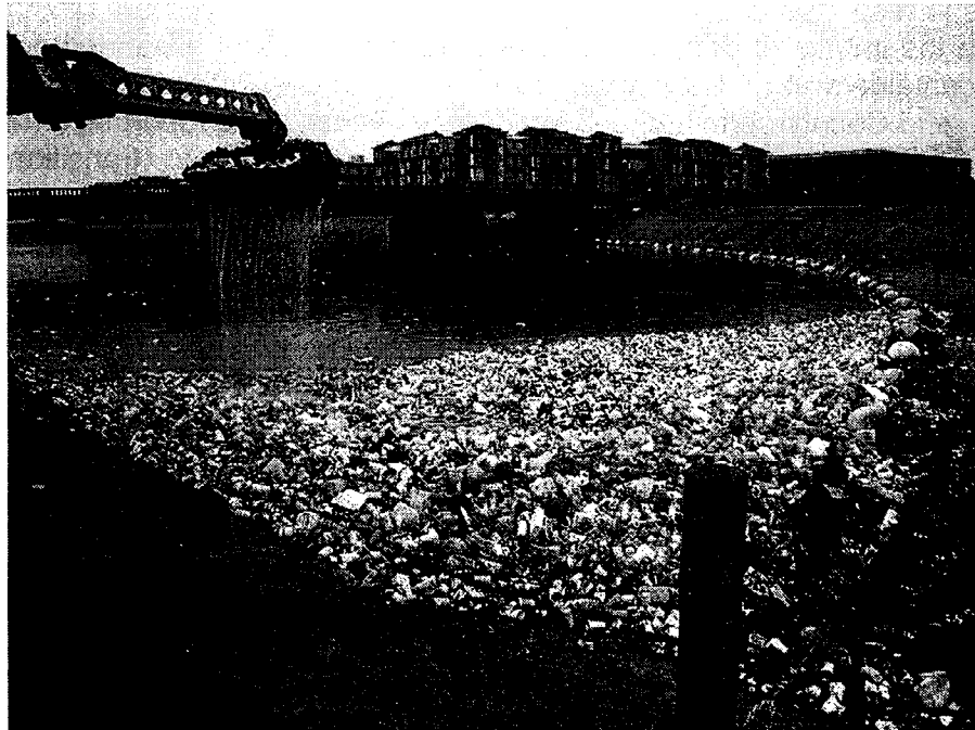
Figure 1 – Expanded Polystyrene Cups And Other Plastic Trash Captured In The Los Angeles River Debris Net
