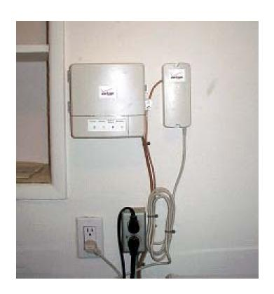
Power Supply and Battery Back-up
