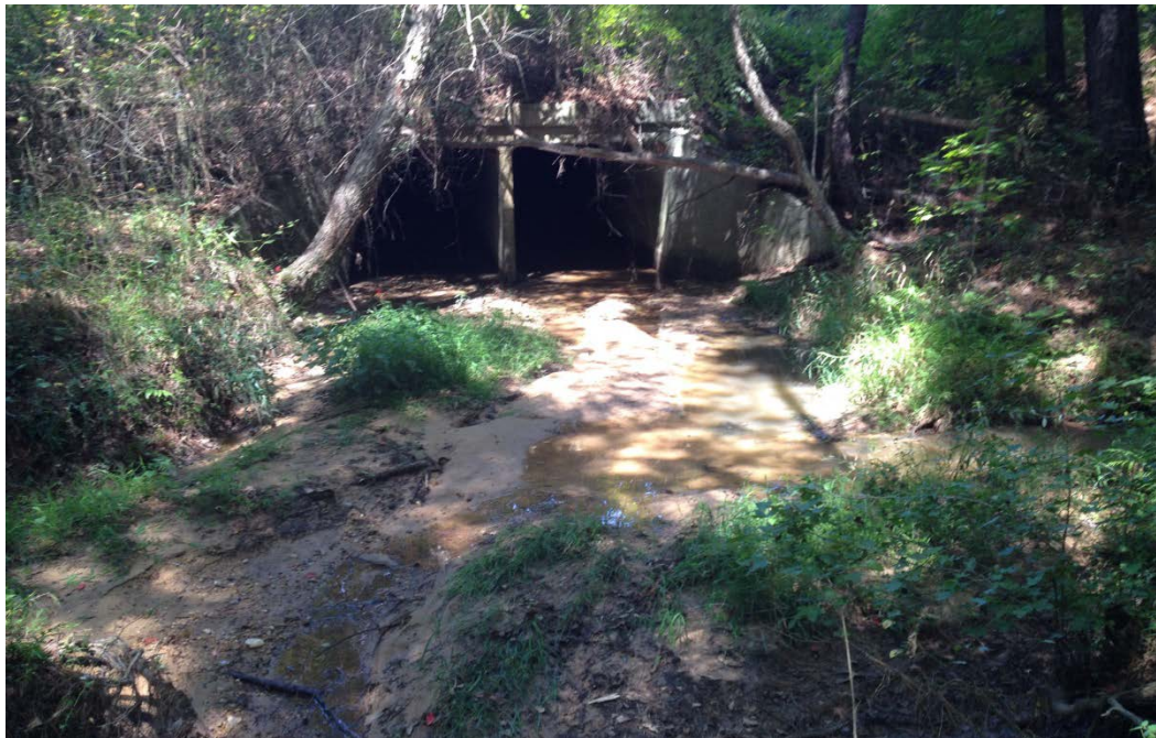
Photo 4: Stream Channel looking north at outlet culvert below US-1.
