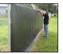
Fence Specifications: 1. Chain Link Fence to be 60" in height, galvanized, with safety edge on top. 2. Acoustifence Specifications 3. Acoustii Fence installed per manufacturers recommendations. See specifications below: a. Acoustical Rating: STC 28 / OITC 22 b. Acoustical test per ASTM E90-04, ASTM E413-04, ASTM E2235-04 :. Size: 6 ft. x 30 ft. x 0.125 in. =  $180 \text{ ft}^2$
