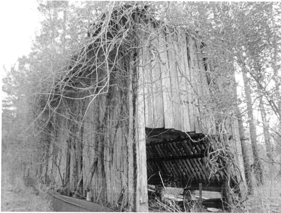
Barn along Bynum Ridge Road
