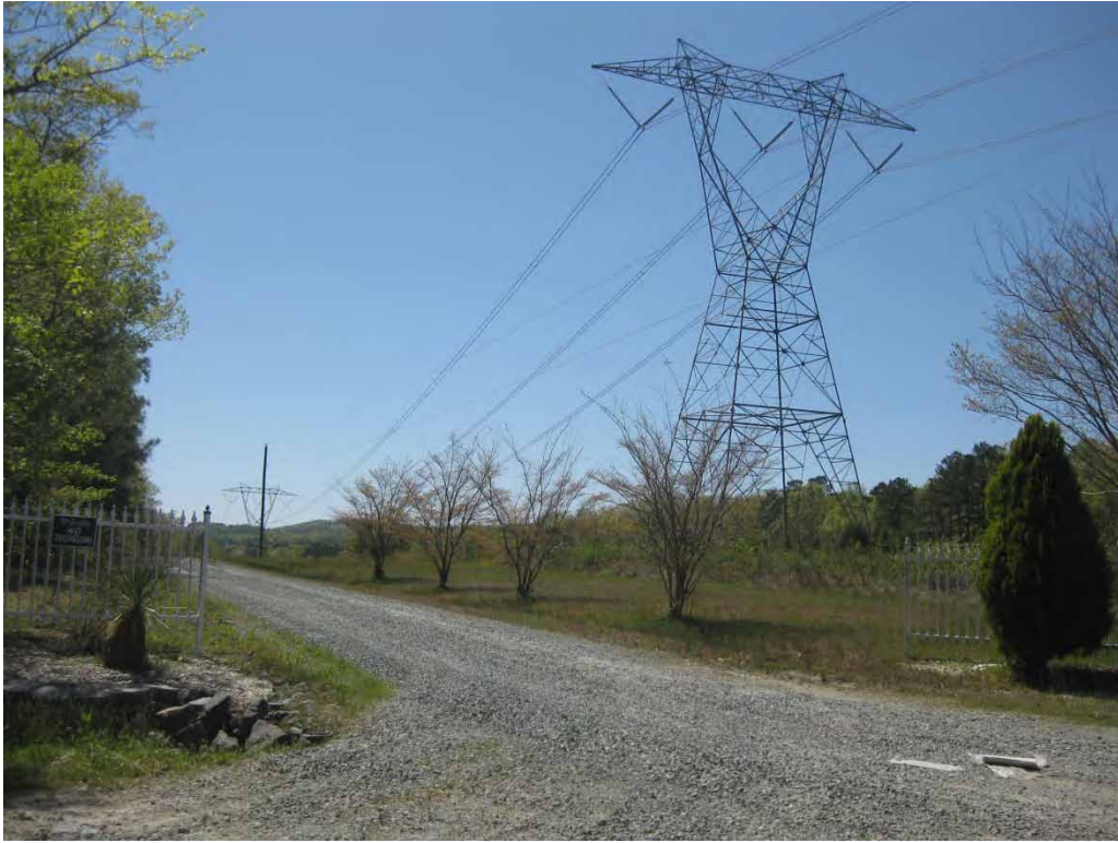
Transmission Line Easement Near the Site
