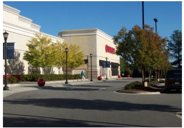
Figure 17: Example of Break In Façade Massing. Note both horizontal setback variation (entrance) and vertical steps to break up the roofline.
