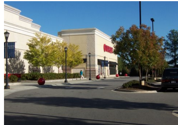
Figure 19: Example of Break In Façade Massing. Note both horizontal setback variation (entrance) and vertical steps to break up the roofline.
