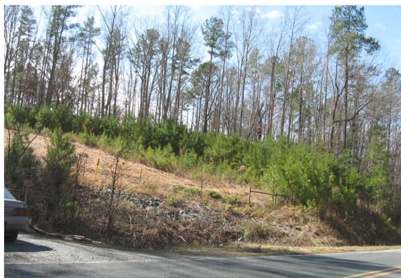
▲ North-facing R-O-W slope to Andrews Store Road. Lot 20 (pine trees).
