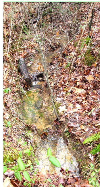
Upstream from culvert 2 (between lots 14 & 15). ▼
