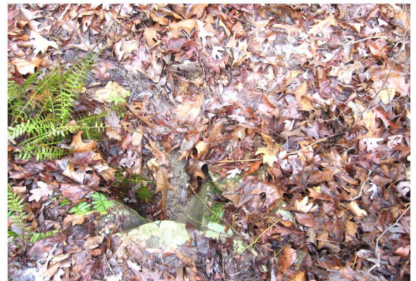
▲ Two views of storm water runoff to culvert 3. (Open space between lots 11 & 13.)
