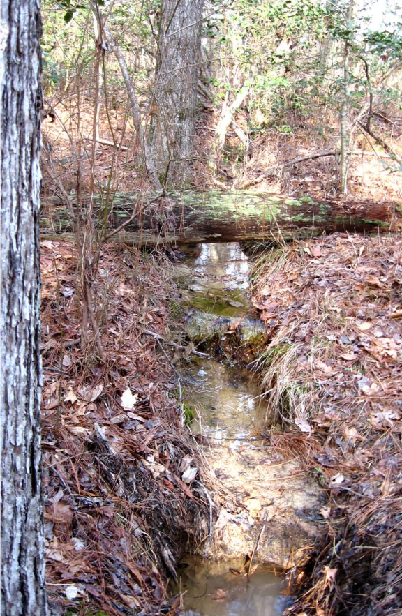
Upstream from culvert 4. Lot 21.▲
